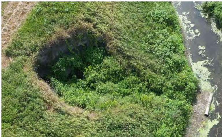
Figure 6. Collapsed Tile into the Main Open Ditch
