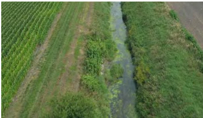
Picture #7: Sediment and Vegetation Accumulation along the Open Ditch in Section 30 of Sterling Township
