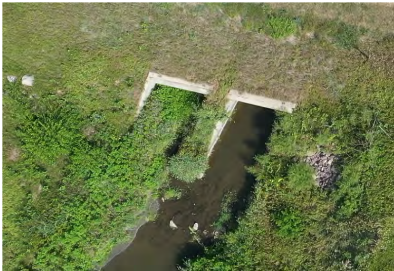
Figure 9. Constricted Road Crossing on 119th Street on the Main Open Ditch
