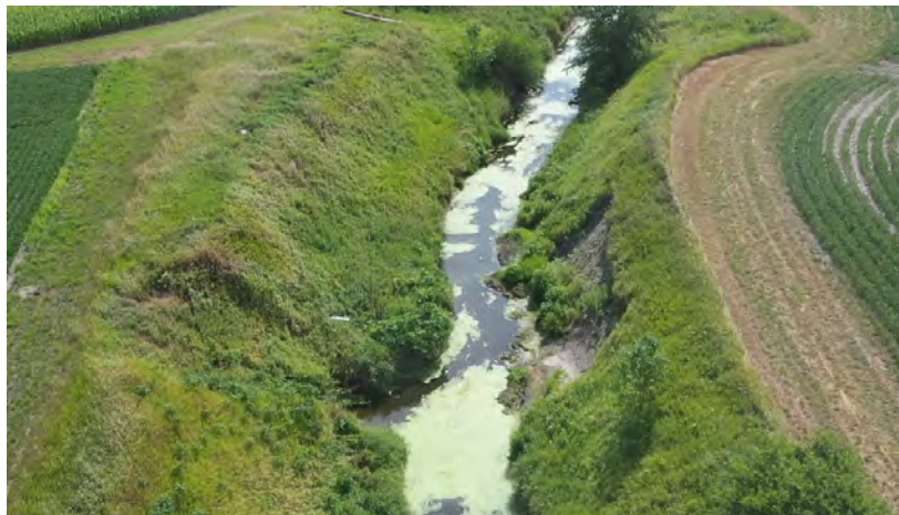
Figure 7. Sloughing along open ditch in the Southeast Quarter of Section 18 in Sterling Township
