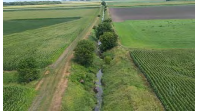
Picture #6: Heavy Vegetation along ditch Banks and Unprotected Tile Outlets in Section 30 of Sterling Township
