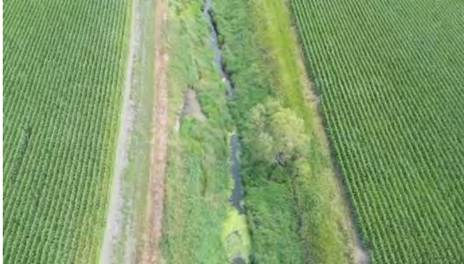
Picture #5: Sloughing along Ditch Bank in Section 30 of Sterling Township
