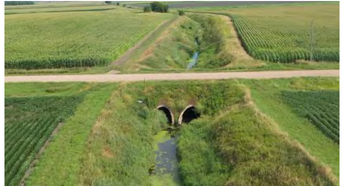
Picture #4: Sediment and Vegetation Accumulation in Culvert Crossing along 108 th Street in Section 30 of Sterling Township
