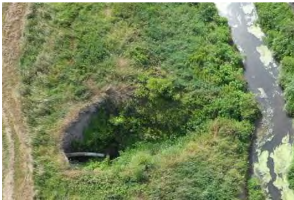
Picture #15: Collapsed Tile in Section 18 of Sterling Township
