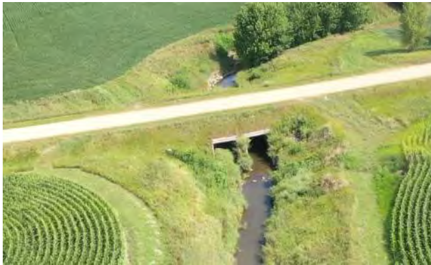
Picture #21: Culvert Crossing with 119 th Street in Section 17 of Sterling Township, Heavy Sediment Deposition in West Box Culvert
