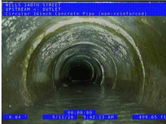
HUEPER BRANCH OUTLET (US) UPSTREAM_668641c2-2fcd-4986-bc7f-fc9da7c5b44e_20200911_100250_705.jpg, 00:17:17, 499.64ft Water Level, 30% of the vertical dimension / LOCATER DEPTH 5'6"
