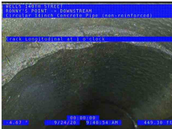
RONNY'S POINT (DS) DOWNSTREAM_43655d47-7dbe-4540-85a6-a4e5d6c65c2d_20200924_100313_088.jpg, 00:09:33, 449.30ft Crack Longitudinal at 1 o'clock
