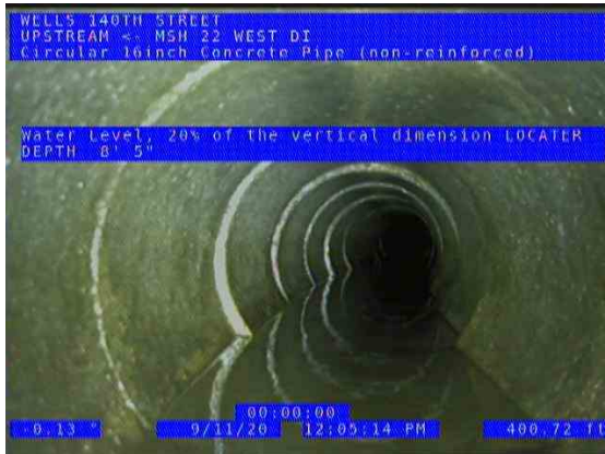
MSH 22 WEST (US) UPSTREAM_d02004f2-de31-45b6-9842-19acd4368742_2020 0911_122540_883.jpg, 00:29:57, 400.72ft Water Level, 20% of the vertical dimension / LOCATER DEPTH 8' 5"
