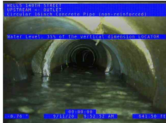
HUEPER BRANCH OUTLET (US) UPSTREAM_044baaa9-b90c-4020-a1d1-4f5517bcfee3_2020 0911_101320_023.jpg, 00:21:53, 641.50ft Water Level, 35% of the vertical dimension / LOCATOR DEPTH 7'0"
