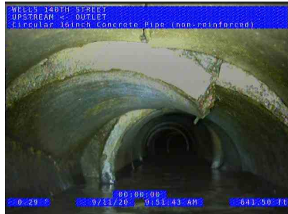
HUEPER BRANCH OUTLET (US) UPSTREAM_ff8b467a-fca3-4e00-b752-e3d13ae92a85_20200 911_101210_495.jpg, 00:21:16, 637.92ft Broken from 11 o'clock to 1 o'clock, length: 10inch, intruding: 4inch / MULTIPLE TILE FAILING
