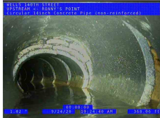
RONNY'S POINT (US) UPSTREAM_bde5e63e-16d8-4939-ad0f-a879f5b9c353_2020 0924_104658_501.jpg, 00:15:01, 368.81ft Joint Separated Large, 2Inch / COVERED WITH CLAY AT SEAM
