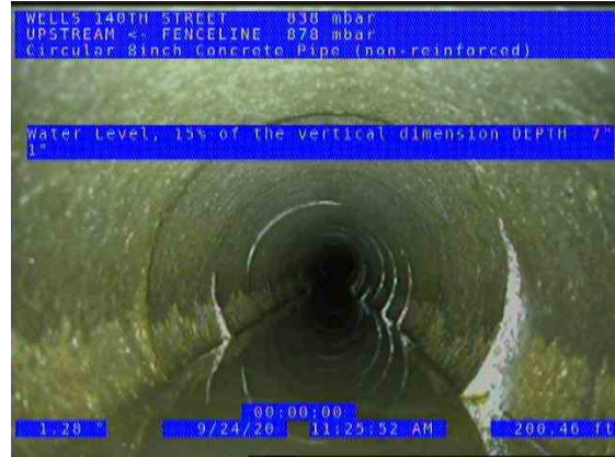
FENCELINE POINT (US) UPSTREAM_75c6ef38-44ed-4421-a65c-ed163a308056_2020 0924_114811_441.jpg, 00:06:06, 200.46ft Water Level, 15% of the vertical dimension / DEPTH 7" 1"
