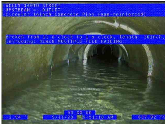
HUEPER BRANCH OUTLET (US) UPSTREAM_23cf957b-cf6b-479f-abcd-5523457cbf2c_202009 11_101137_455.jpg, 00:21:16, 637.92ft Broken from 11 o'clock to 1 o'clock, length: 10inch, intruding: 4inch / MULTIPLE TILE FAILING
