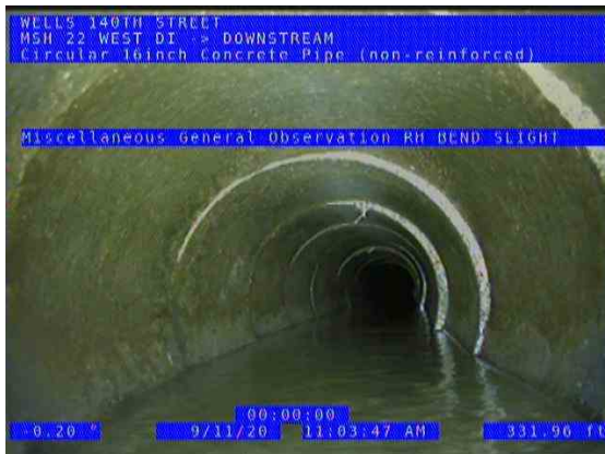
MSH 22 WEST DI (DS) DOWNSTREAM_4a801da2-e5af-4aed-bdac-494b294579a7_2 0200911_112414_303.jpg, 00:15:08, 331.96ft Miscellaneous General Observation / RH BEND SLIGHT
