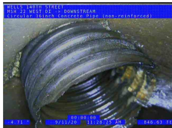
MSH 22 WEST DI (DS) DOWNSTREAM_b861e18b-0801-442d-b114-d78911b5e7a3_20200911_114852_430.jpg, 00:29:12, 846.78ft Tap Break-in Activity at 2 o'clock, dia/height: 6inch
