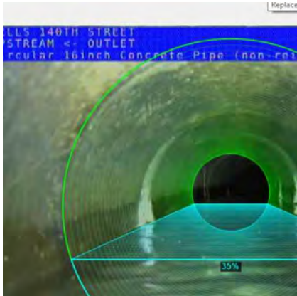
HUEPER BRANCH OUTLET (US) UPSTREAM_62ef70e4-26b6-430d-8e0b-3b5aa36e61d0_2020 0911_093937_252.jpg, 00:04:36, 68.26ft Water Level, 35% of the vertical dimension
