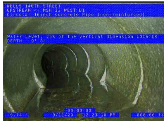
MSH 22 WEST (US) UPSTREAM_b24caf9b-a3f2-43ed-a966-91550912e4b8_20200911_124336_737.jpg, 00:29:57, 808.66ft Water Level, 25% of the vertical dimension / LOCATER DEPTH 9' 8"
