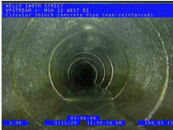
MSH 22 WEST (US) UPSTREAM_e9891966-3569-4c24-9a00-47efb314d858_2020 0911_122020_432.jpg, 00:29:57, 198.84ft Water Level, 15% of the vertical dimension / LOCATER DEPTH 7' 6" there is a hump in pipe here
