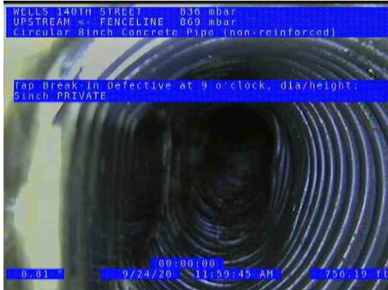
FENCELINE POINT (US) UPSTREAM_06da4976-ea3c-4f97-a795-b85963c21597_2020 0924_122204_841.jpg, 00:26:06, 756.19ft Tap Break-In Defective at 9 o'clock, dia/height: 5inch / PRIVATE
