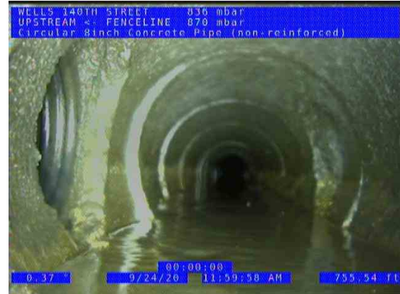
FENCELINE POINT (US) UPSTREAM_680b6eb1-c1be-4a4b-b9ce-f67bf88ebe9d_2020 0924_122218_272.jpg, 00:26:06, 756.19ft Tap Break-In Defective at 9 o'clock, dia/height: 5inch / PRIVATE
