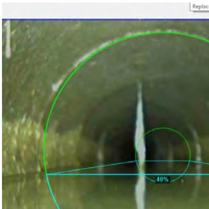
FENCELINE POINT (US) UPSTREAM_d9dda0ad-a71a-4077-b267-19f6f7f21b3f_20200 924_121050_774.jpg, 00:23:37, 899.51ft Water Level, 40% of the vertical dimension / DEPTH 4'
