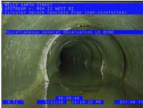
MSH 22 WEST (US) UPSTREAM_e93e03b4-3f1d-4f0e-902f-26ab7cf556f0_20200911_124441_709.jpg, 00:29:57, 837.97ft Miscellaneous General Observation / LH BEND
