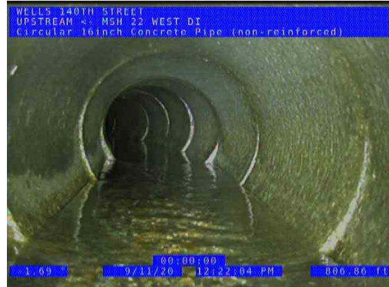
MSH 22 WEST (US) UPSTREAM_384bd8e1-30f5-43c3-8b31-ef7d30c03714_20200911_124231_007.jpg, 00:29:57, 806.86ft Miscellaneous General Observation / LH BEND
