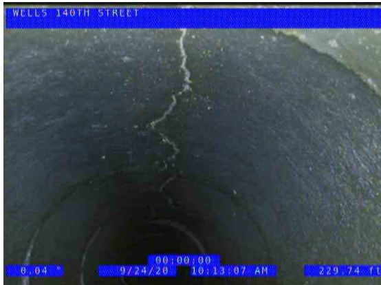
RONNY'S POINT (US) UPSTREAM_0e1bc8c6-9bd7-473f-af5c-a9a4c50491df_2020 0924_103525_526.jpg, 00:08:16, 229.74ft Crack Longitudinal at 12 o'clock / END OF A FEW BAD TILE
