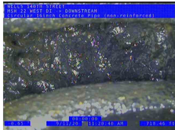
MSH 22 WEST DI (DS) DOWNSTREAM_225ea995-58b2-4ca1-a784-ad9921b512bd_ 20200911_114107_242.jpg, 00:24:58, 717.12ft Joint Offset Large, 2Inch / SEVERAL MISALIGNED TILE
