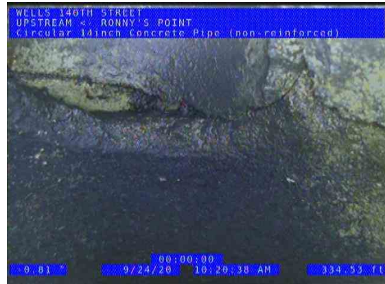
RONNY'S POINT (US) UPSTREAM_1f801f72-8a5b-4421-b018-c4ccc3c00d65_20200924_104256_049.jpg, 00:12:16, 336.39ft Tap Break-in Activity at 3 o'clock, dia/height: 6inch / CLAY BACK TO THE RIGHT
