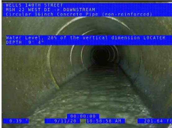
MSH 22 WEST DI (DS) DOWNSTREAM_395dad04-3482-4912-964a-9d9d7e94acc8_ 20200911_111925_370.jpg, 00:10:41, 201.64ft Water Level, 20% of the vertical dimension / LOCATER DEPTH 9' 4"
