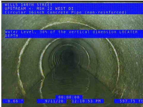
MSH 22 WEST (US) UPSTREAM_0b44f384-49e4-4401-99b7-7fa61ddf8d73_20200911_123120_181.jpg, 00:29:57, 597.75ft Water Level, 30% of the vertical dimension / LOCATER DEPTH
