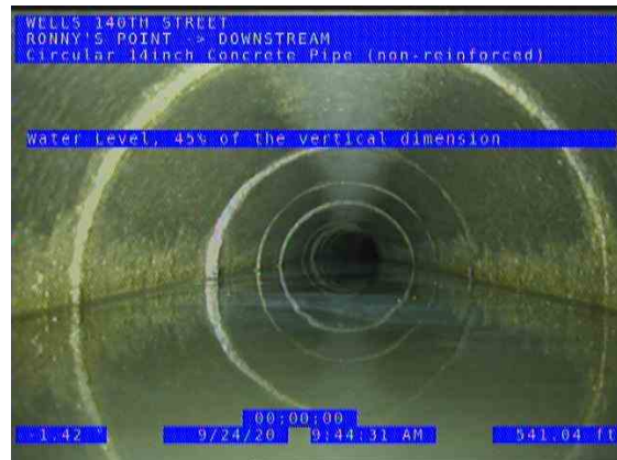
RONNY'S POINT (DS) DOWNSTREAM_ab052775-cad1-4094-9ee9-62205d2e6e09_ 20200924_100649_467.jpg, 00:11:58, 541.04ft Water Level, 45% of the vertical dimension
