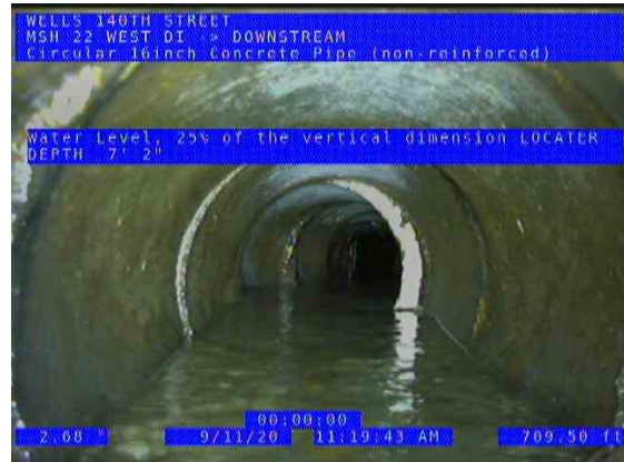
MSH 22 WEST DI (DS) DOWNSTREAM_fe720a86-5251-417d-a5cc-0053f7799f50_20 200911_114010_165.jpg, 00:24:30, 709.50ft Water Level, 25% of the vertical dimension / LOCATER DEPTH 7' 2"
