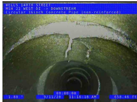
MSH 22 WEST DI (DS) DOWNSTREAM_b0df0b05-c367-41bb-a07f-acacdd78ac5d_2 0200911_113645_469.jpg, 00:22:50, 662.22ft Broken at 12 o'clock, length: 2inch / 1 TILE BROKEN SEVERAL CRACKED
