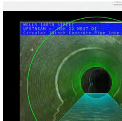
MSH 22 WEST (US) UPSTREAM_014d88d7-a137-4498-ac89-7eb22664e7f4_2020 0911_121900_996.jpg, 00:29:57, 198.84ft Water Level, 15% of the vertical dimension / LOCATER DEPTH 7' 6" there is a hump in pipe here
