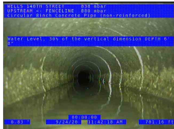
FENCELINE POINT (US) UPSTREAM_be5c8ddc-d576-4cde-93c1-13728a6ceff7_20200 924_120437_917.jpg, 00:17:52, 701.16ft Water Level, 30% of the vertical dimension / DEPTH 6' 8"
