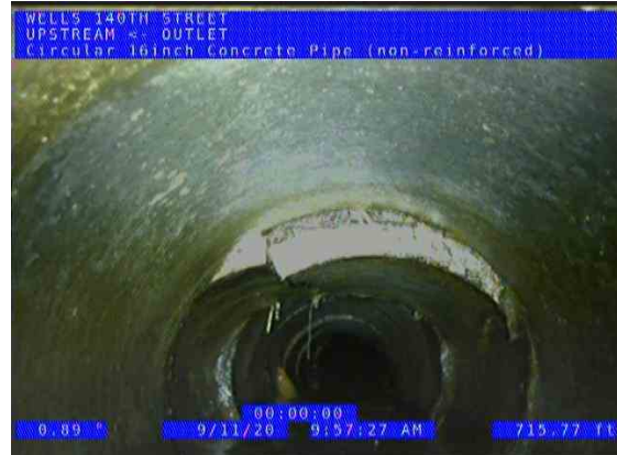
HUEPER BRANCH OUTLET (US) UPSTREAM_120b2eca-5ce9-4ee4-b1d5-d46d0b1c7bf3_2020 0911_101754_365.jpg, 00:24:59, 713.21ft Broken from 11 o'clock to 1 o'clock, length: 10inch, intruding: 4inch / COLLAPSING
