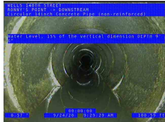
RONNY'S POINT (DS) DOWNSTREAM_ef1f15d3-9a07-454a-8dbd-5363770222ad_2 0200924_095148_266.jpg, 00:01:58, 100.59ft Water Level, 15% of the vertical dimension / DEPTH 9' 6"
