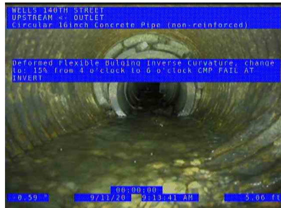
HUEPER BRANCH OUTLET (US) UPSTREAM_4c48e0ef-33d7-4455-a360-c3de5c30cc74_2020 0911_093408_971.jpg, 00:00:17, 5.06ft Deformed Flexible Bulging Inverse Curvature, change to: 15% from 4 o'clock to 6 o'clock / CMP FAIL AT INVERT
