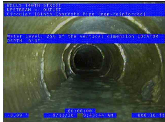
HUEPER BRANCH OUTLET (US) UPSTREAM_12813a7a-e575-4610-8c47-6ae36065cfbf_20200911_100911_594.jpg, 00:20:00, 600.10ft Water Level, 25% of the vertical dimension / LOCATER DEPTH 6'6"
