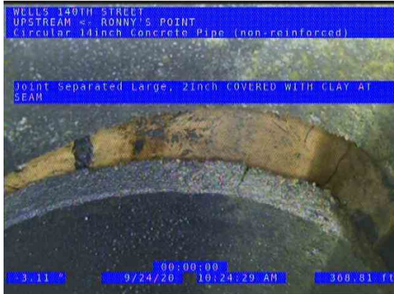
RONNY'S POINT (US) UPSTREAM_bb63fa9a-0620-4617-a6c9-6abe49611074_2020 0924_104647_593.jpg, 00:15:01, 368.81ft Joint Separated Large, 2Inch / COVERED WITH CLAY AT SEAM
