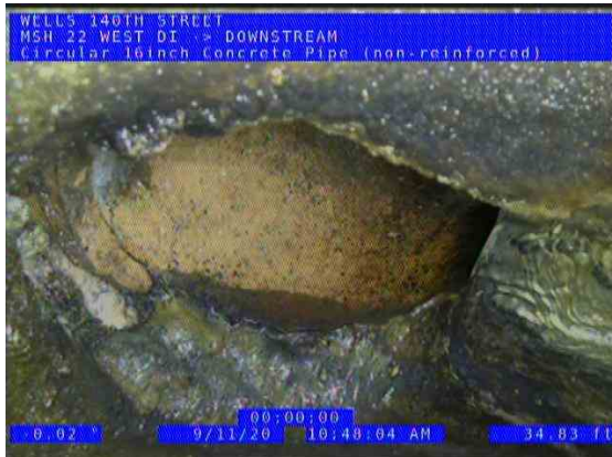
MSH 22 WEST DI (DS) DOWNSTREAM_c14a6d1d-11d1-463b-99f4-fa088e9b1db4_2 0200911_110831_608.jpg, 00:03:09, 35.49ft Tap Break-in Activity at 3 o'clock, dia/height: 5inch / CLAY CONNECTION
