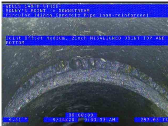
RONNY'S POINT (DS) DOWNSTREAM_bc74da77-9c9f-4795-a618-f5af7dfec002_20 200924_095611_542.jpg, 00:05:04, 297.03ft Joint Offset Medium, 2Inch / MISALIGNED JOINT TOP AND BOTTOM
