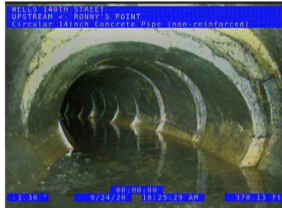
RONNY'S POINT (US) UPSTREAM_57e8f55f-f40e-4120-8ab8-2ff05dc94e57_202009 24_104747_018.jpg, 00:15:27, 370.14ft Miscellaneous Shape or Size Change, dia/height: 12inch / FAILING
