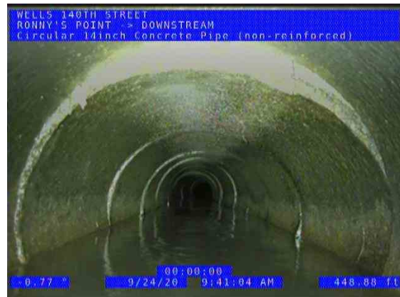
RONNY'S POINT (DS) DOWNSTREAM_7c744c2b-6155-446f-9fbd-11bfa932c5ba_20200924_100322_263.jpg, 00:09:33, 449.30ft Crack Longitudinal at 1 o'clock
