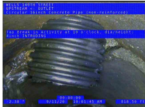
HUEPER BRANCH OUTLET (US) UPSTREAM_493fb134-c9a4-4a87-8907-f65ebaed01c7_2020 0911_102212_412.jpg, 00:29:02, 818.50ft Tap Break-in Activity at 10 o'clock, dia/height: 4inch / INTRUDING, COLLAPSING IN THE PRIVATE TILE
