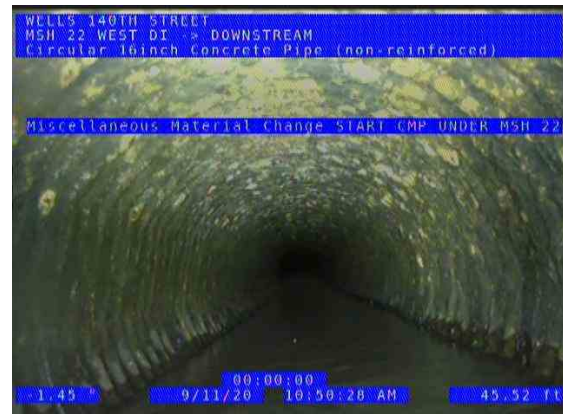
MSH 22 WEST DI (DS) DOWNSTREAM_feb5b991-4280-4fae-9e94-9756aeab935e_2 0200911_111055_659.jpg, 00:05:00, 45.89ft Miscellaneous Material Change / START CMP UNDER MSH 22
