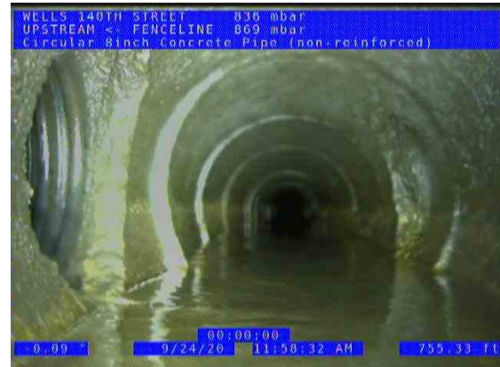
FENCELINE POINT (US) UPSTREAM_037e6d6c-d017-4ede-b073-6a55621c08f5_2020 0924_122051_591.jpg, 00:26:06, 757.30ft Tap Break-in Activity at 3 o'clock, dia/height: 5inch / PRIVATE
