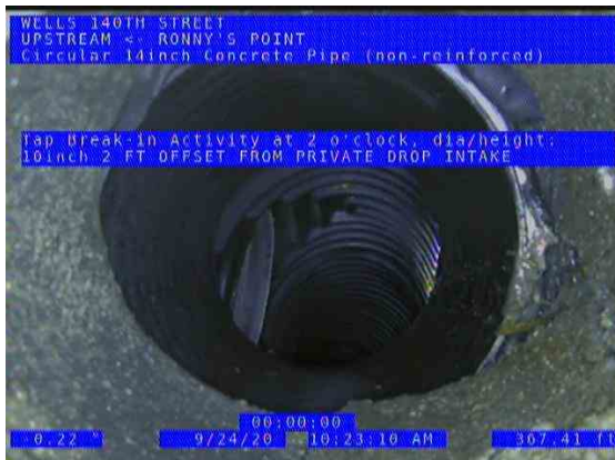
RONNY'S POINT (US) UPSTREAM_b2c5559d-1751-4e12-a06b-f65eda491a81_20200924_104528_821.jpg, 00:14:03, 367.41ft Tap Break-in Activity at 2 o'clock, dia/height: 10inch / 2 FT OFFSET FROM PRIVATE DROP INTAKE
