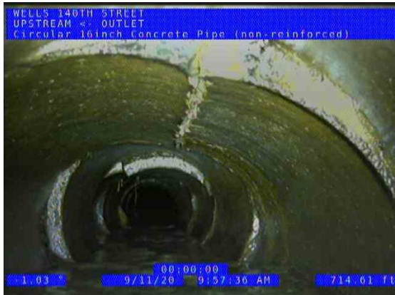
HUEPER BRANCH OUTLET (US) UPSTREAM_d92daa52-41f5-40c7-a997-ffe8c7b5df8_202009 11_101804_347.jpg, 00:24:59, 713.21ft Broken from 11 o'clock to 1 o'clock, length: 10inch, intruding: 4inch / COLLAPSING
