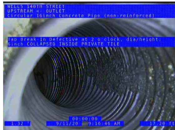
HUEPER BRANCH OUTLET (US) UPSTREAM_ce0e5e53-6a12-49ac-a67c-c8c695227b42_2020 0911_093713_691.jpg, 00:01:35, 17.36ft Tap Break-In Defective at 2 o'clock, dia/height: 6inch / COLLAPSED INSIDE PRIVATE TILE
