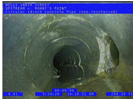
RONNY'S POINT (US) UPSTREAM_c8a3e2e7-f3c8-41d9-af15-b246e8f881b5_20200 924_103849_134.jpg, 00:10:02, 296.31ft Tap Break-in Activity at 3 o'clock, dia/height: 8inch / RUNS UP TO THE NORTH
