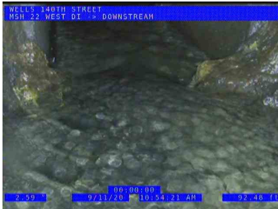
MSH 22 WEST DI (DS) DOWNSTREAM_f5824195-cfad-4458-b205-25eb10b966a4_2 0200911_111448_403.jpg, 00:07:57, 92.48ft Infiltration Dripper Joint from 4 o'clock to 8 o'clock, within 8 inch / SOIL CONSISTANTLY IN JOINTS
