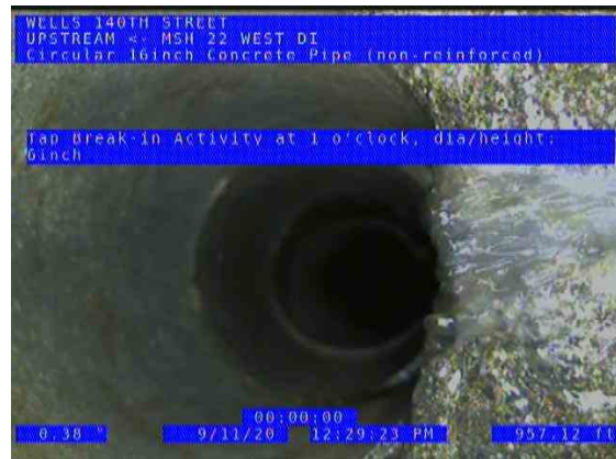
MSH 22 WEST (US) UPSTREAM_e2cf924a-5df1-4f93-9ccd-e9851e0f23c1_20200911_124950_262.jpg, 00:29:57, 957.12ft Tap Break-in Activity at 1 o'clock, dia/height: 6inch
