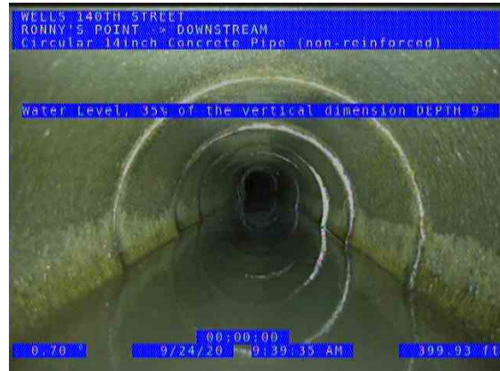
RONNY'S POINT (DS) DOWNSTREAM_6d0e21a5-179f-4729-9fba-ecc14bd805fe_20200924_100153_667.jpg, 00:08:26, 399.93ft Water Level, 35% of the vertical dimension / DEPTH 9' 3"
