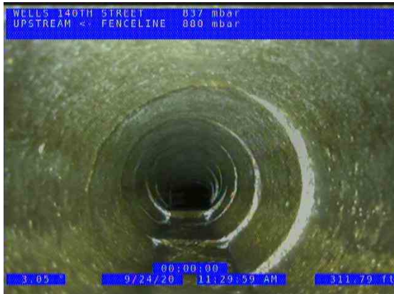
FENCELINE POINT (US) UPSTREAM_46529899-ff49-47cc-bd4d-410136e5981c_2020 0924_115218_848.jpg, 00:09:00, 311.79ft Water Level, 5% of the vertical dimension / HUMP IN PIPE
