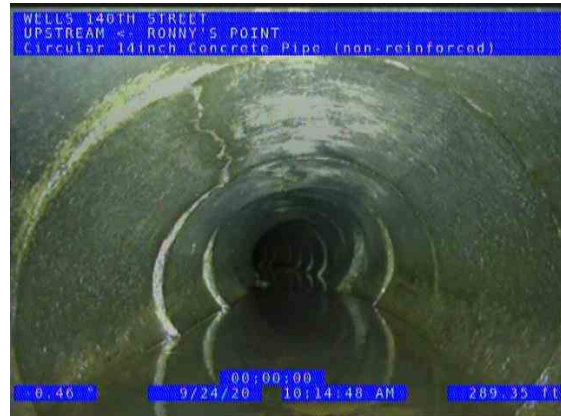
RONNY'S POINT (US) UPSTREAM_6053434c-195f-49ed-bbda-1295638bfaa5_2020 0924_103705_803.jpg, 00:09:24, 289.35ft Broken at 12 o'clock / START OF BROKEN TILE DEPTH 5' 9"
