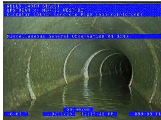
MSH 22 WEST (US) UPSTREAM_ffdf3937-b51f-4605-afd6-8f23b4b81b0a_20200911_123611_270.jpg, 00:29:57, 699.80ft Miscellaneous General Observation / RH BEND
