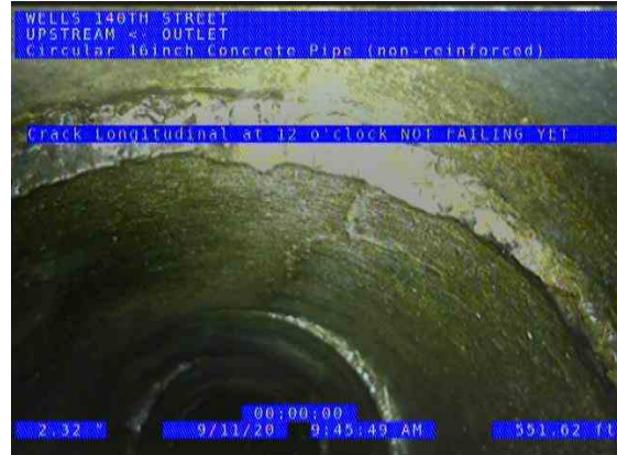
HUEPER BRANCH OUTLET (US) UPSTREAM_e6ab26fa-49b3-489f-97b9-0b05a3cfd5c_20200911_100617_103.jpg, 00:18:46, 551.62ft Crack Longitudinal at 12 o'clock / NOT FAILING YET
