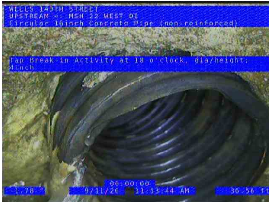
MSH 22 WEST (US) UPSTREAM_cb150d80-c8cd-4664-838c-e87b292d293e_2020 0911_121410_651.jpg, 00:29:57, 36.56ft Tap Break-in Activity at 10 o'clock, dia/height: 4inch
