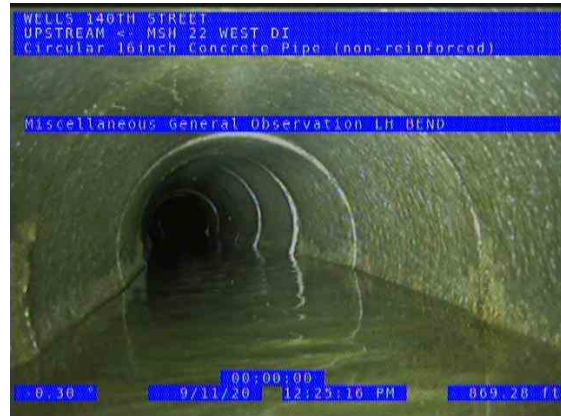
MSH 22 WEST (US) UPSTREAM_0db4eeb7-56b8-4d53-bf95-725b697fb9ec_20200911_124543_057.jpg, 00:29:57, 869.28ft Miscellaneous General Observation / LH BEND
