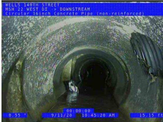
MSH 22 WEST DI (DS) DOWNSTREAM_c175e4ec-5a87-44ca-aec0-985ab2599884_20200911_110546_714.jpg, 00:01:08, 17.52ft Tap Break-In Defective at 2 o'clock, dia/height: 4inch / COLLAPSED OUTSIDE OF CONCRETE
