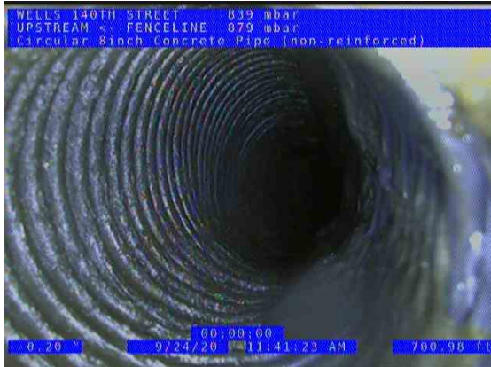
FENCELINE POINT (US) UPSTREAM_5283c6b1-3c85-4e7c-80f1-634038d44782_2020 0924_120344_062.jpg, 00:17:23, 700.98ft Tap Break-in Activity at 2 o'clock, dia/height: 5inch / PUT IN 2015-PRIVATE
