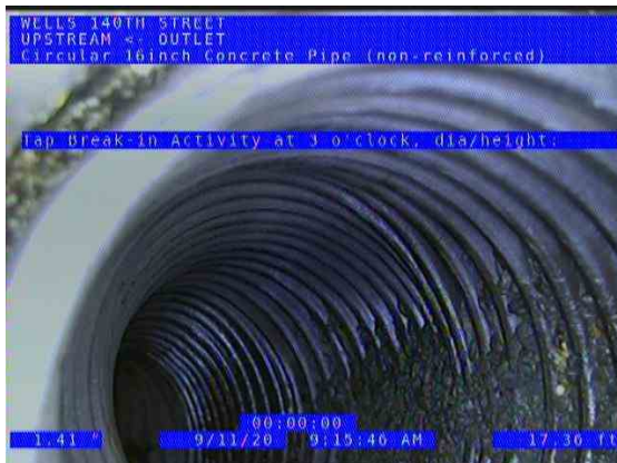
HUEPER BRANCH OUTLET (US) UPSTREAM_501d19e1-907c-490a-a78d-7d8bd28d6a86_202 00911_093614_123.jpg, 00:01:35, 17.36ft Tap Break-In Defective at 2 o'clock, dia/height: 6inch / COLLAPSED INSIDE PRIVATE TILE
