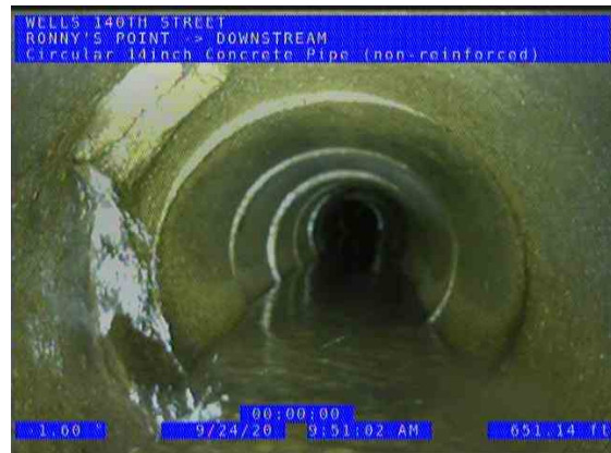
RONNY'S POINT (DS) DOWNSTREAM_6f94e5b0-7713-420b-84cb-a15ea3dd3c85_2 0200924_101320_685.jpg, 00:15:30, 651.68ft Tap Break-in Activity at 10 o'clock, dia/height: 5inch / 5" CLAY
