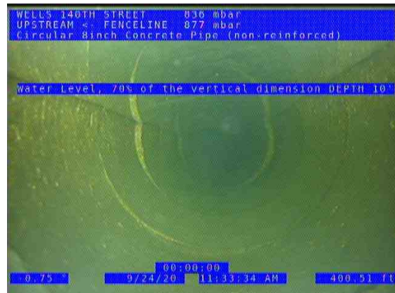
FENCELINE POINT (US) UPSTREAM_d1661635-ae2c-4e8b-931e-0a02994c9979_20200924_115554_309.jpg, 00:11:04, 400.51ft Water Level, 70% of the vertical dimension / DEPTH 10'
