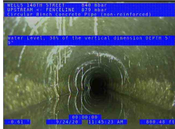
FENCELINE POINT (US) UPSTREAM_979bc4a1-d85f-428f-b458-a797c7bcc3ad_20200 924_120743_508.jpg, 00:20:31, 800.47ft Water Level, 30% of the vertical dimension / DEPTH 5' 9"
