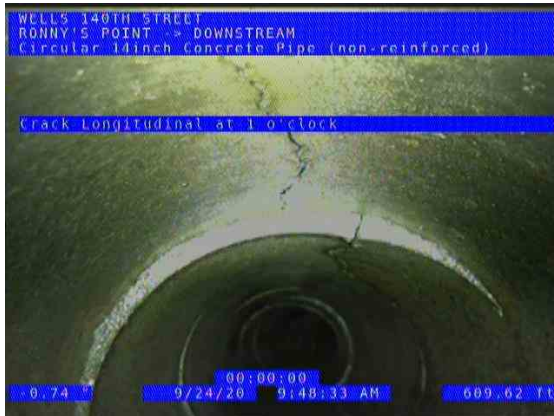
RONNY'S POINT (DS) DOWNSTREAM_6de5e123-def9-4616-82cc-5593a249632b_2 0200924_101051_613.jpg, 00:14:02, 609.62ft Crack Longitudinal at 1 o'clock
