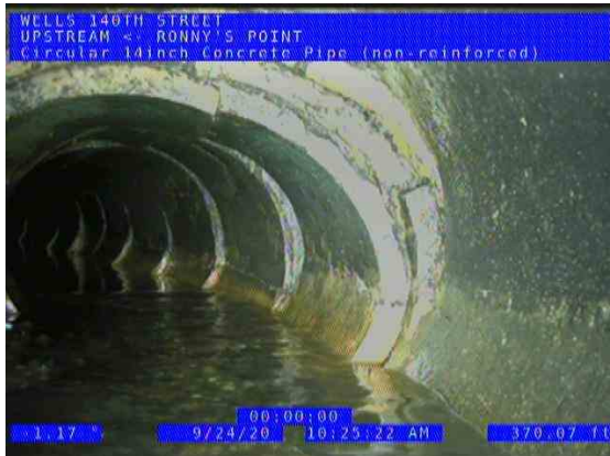
RONNY'S POINT (US) UPSTREAM_604ccbf6-a7a6-4249-9718-82773e2145ec_2020 0924_104740_987.jpg, 00:15:27, 370.14ft Miscellaneous Shape or Size Change, dia/height: 12inch / FAILING
