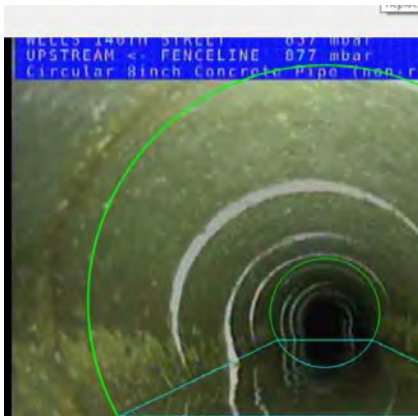
FENCELINE POINT (US) UPSTREAM_7de2b54c-62cd-40f2-afd8-afac93c8a69e_20200 924_120022_579.jpg, 00:15:05, 600.65ft Water Level, 25% of the vertical dimension / DEPTH 8' 4"
