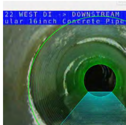
MSH 22 WEST DI (DS) DOWNSTREAM_49e1c3c7-08a6-408c-b13a-300979d90761_20200911_114933_502.jpg, 00:29:33, 846.63ft Water Level, 15% of the vertical dimension / LOCATER DEPTH 7' 4"
