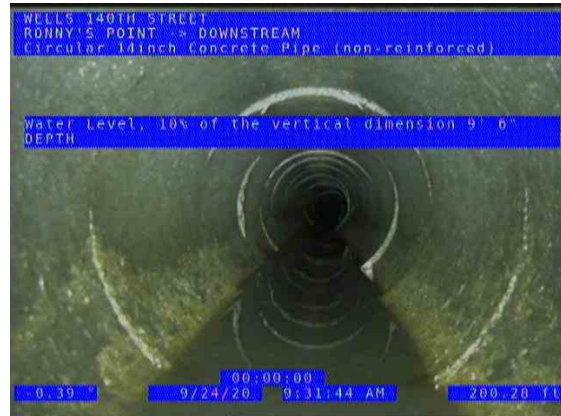
RONNY'S POINT (DS) DOWNSTREAM_950f400f-6c01-4408-96c4-1f058143222b_20 200924_095403_088.jpg, 00:03:29, 200.28ft Water Level, 10% of the vertical dimension / 9' 6" DEPTH
