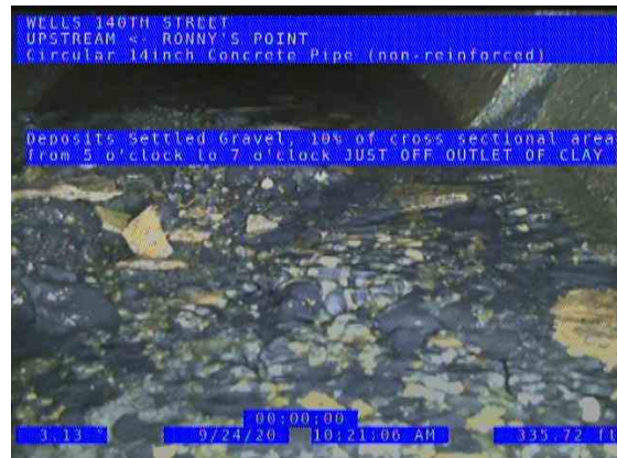
RONNY'S POINT (US) UPSTREAM_fa0b7912-a67b-4285-a6a3-2cd3f7516eb5_2020 0924_104324_336.jpg, 00:12:49, 335.72ft Deposits Settled Gravel, 10% of cross sectional area from 5 o'clock to 7 o'clock / JUST OFF OUTLET OF CLAY
