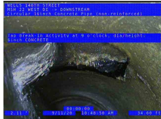
MSH 22 WEST DI (DS) DOWNSTREAM_4239c331-6457-4d58-bb7b-c30842aa8c7b_ 20200911_110918_303.jpg, 00:03:42, 35.50ft Tap Break-in Activity at 9 o'clock, dia/height: 6inch / CONCRETE
