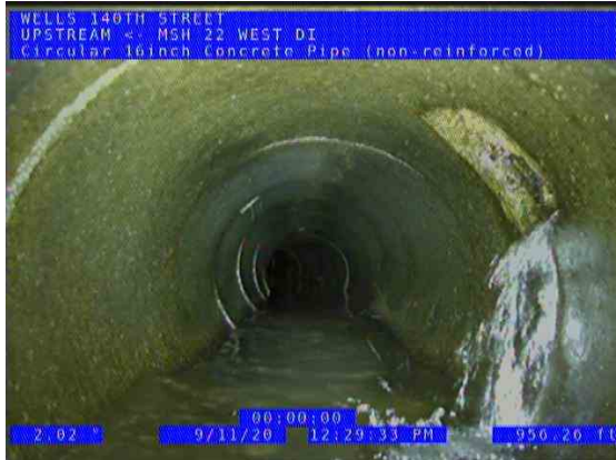
MSH 22 WEST (US) UPSTREAM_6e45c733-1664-4f55-92b2-ad2e1fc85749_2020 0911_125000_166.jpg, 00:29:57, 957.12ft Tap Break-in Activity at 1 o'clock, dia/height: 6inch
