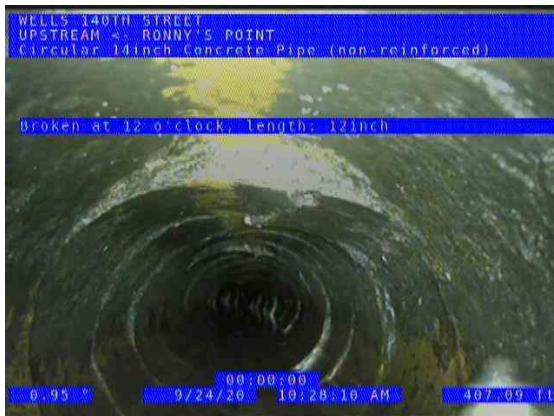
RONNY'S POINT (US) UPSTREAM_e79b1519-cffb-4246-8141-0b242127b4df_20200 924_105028_736.jpg, 00:17:17, 407.09ft Broken at 12 o'clock, length: 12inch
