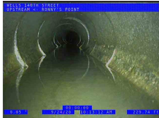
RONNY'S POINT (US) UPSTREAM_39553e5a-45b3-48ca-9860-18def4ea2392_2020 0924_103530_053.jpg, 00:08:16, 229.74ft Crack Longitudinal at 12 o'clock / END OF A FEW BAD TILE
