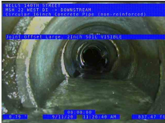
MSH 22 WEST DI (DS) DOWNSTREAM_8cedb893-2e46-458c-9dc5-98feb45ce5c0_20200911_114707_546.jpg, 00:28:46, 837.47ft Joint Offset Large, 2Inch / SOIL VISIBLE
