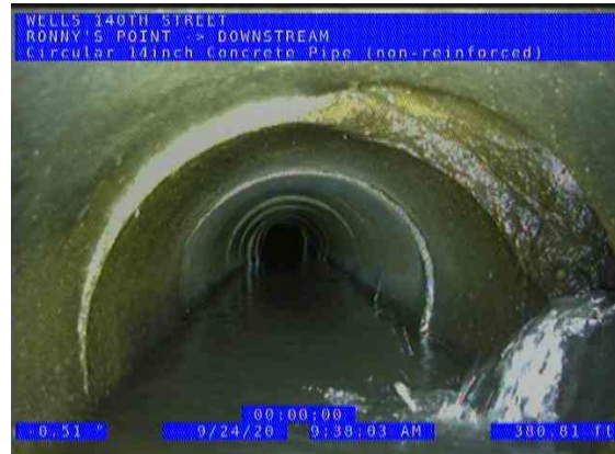
RONNY'S POINT (DS) DOWNSTREAM_b6e2e23b-1056-42be-b9aa-237690aed570_ 20200924_100020_826.jpg, 00:06:56, 382.02ft Tap Break-in Activity at 2 o'clock, dia/height: 8inch / PRIVATE FROM INTAKE TO SOUTH
