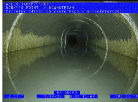
RONNY'S POINT (DS) DOWNSTREAM_2a4bd338-38cb-4dff-819c-dd2ffb2fd2ad_202 00924_095730_039.jpg, 00:05:27, 300.81ft Water Level, 45% of the vertical dimension / 9' 3" DEPTH
