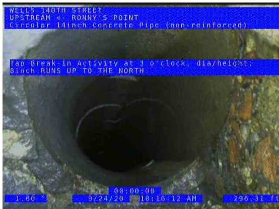
RONNY'S POINT (US) UPSTREAM_c9ad6c2b-abba-43d6-8f98-f6687e889642_2020 0924_103831_240.jpg, 00:10:02, 296.31ft Tap Break-in Activity at 3 o'clock, dia/height: 8inch / RUNS UP TO THE NORTH
