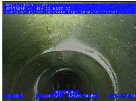
MSH 22 WEST (US) UPSTREAM_8042e241-301e-4f92-acb7-b39acf8c1d2f_20200911_124026_797.jpg, 00:29:57, 770.02ft Crack Longitudinal at 12 o'clock, length: 1inch / SEVERAL
