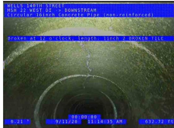
MSH 22 WEST DI (DS) DOWNSTREAM_e18954db-a9d4-4ba0-b48b-64a52c9a7015_ 20200911_113503_040.jpg, 00:21:20, 632.72ft Broken at 12 o'clock, length: 1inch / 2 BROKEN TILE LOCATER DEPTH 8' 2"
