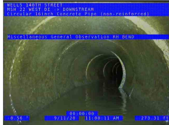
MSH 22 WEST DI (DS) DOWNSTREAM_1dcfe3cb-e873-4dba-b054-ba3f56f4a64a_20 200911_112038_251.jpg, 00:11:47, 279.82ft Miscellaneous General Observation / RH BEND LOCATER DEPTH 10' 4"
