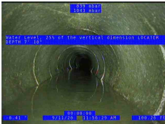
MSH 22 WEST (US) UPSTREAM_5d5a549e-b193-43d7-8cce-99789ad4464c_2020 0911_121655_486.jpg, 00:29:57, 100.26ft Water Level, 25% of the vertical dimension / LOCATER DEPTH 7' 10"
