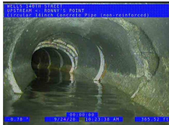
RONNY'S POINT (US) UPSTREAM_1a5df952-1228-47c1-89f2-3fd578278d69_20200924_104556_546.jpg, 00:14:03, 367.41ft Tap Break-in Activity at 2 o'clock, dia/height: 10inch / 2 FT OFFSET FROM PRIVATE DROP INTAKE
