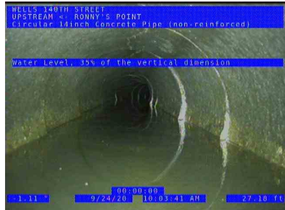
RONNY'S POINT (US) UPSTREAM_c44aad47-09bf-4aa0-a196-fe6b5fd4003b_20200 924_102559_853.jpg, 00:01:27, 27.18ft Water Level, 35% of the vertical dimension
