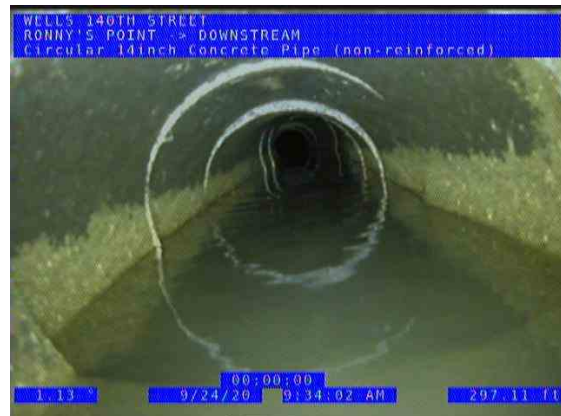
RONNY'S POINT (DS) DOWNSTREAM_5ad2dfc0-9d05-4da9-aa06-d874e3514351_2 0200924_095619_945.jpg, 00:05:04, 297.03ft Joint Offset Medium, 2Inch / MISALIGNED JOINT TOP AND BOTTOM
