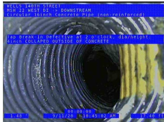
MSH 22 WEST DI (DS) DOWNSTREAM_e12a6a6b-80d2-4101-aaf7-940b6f3b7361_2 0200911_110529_961.jpg, 00:01:08, 17.52ft Tap Break-In Defective at 2 o'clock, dia/height: 4inch COLLAPED OUTSIDE OF CONCRETE
