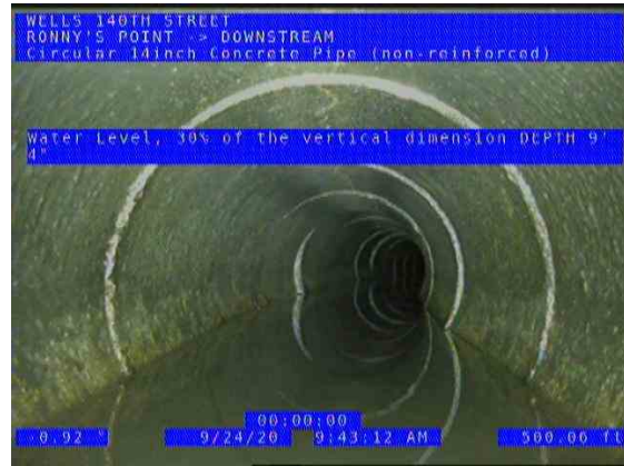
RONNY'S POINT (DS) DOWNSTREAM_80d1b92c-2c63-4000-b9fa-c15abce6db7e_2 0200924_100530_968.jpg, 00:11:07, 500.06ft Water Level, 30% of the vertical dimension / DEPTH 9' 4"
