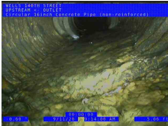
HUEPER BRANCH OUTLET (US) UPSTREAM_3c1e7256-2f41-4754-b1b6-1944c65ee355_2020 0911_093427_845.jpg, 00:00:17, 5.06ft Deformed Flexible Bulging Inverse Curvature, change to: 15% from 4 o'clock to 6 o'clock / CMP FAIL AT INVERT
