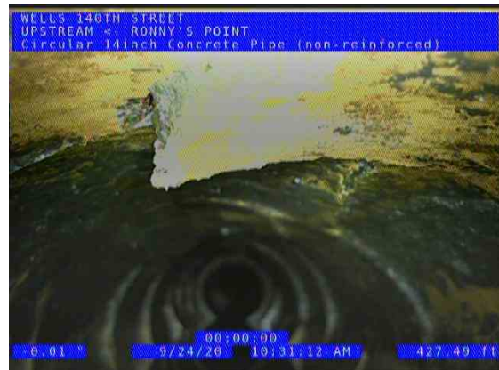
RONNY'S POINT (US) UPSTREAM_89be9b19-dbf9-4655-96fd-f51179d77125_20200924_105330_344.jpg, 00:19:08, 427.49ft Miscellaneous Survey Abandoned / UNABLE TO CONTINUE, BROKEN TILE
