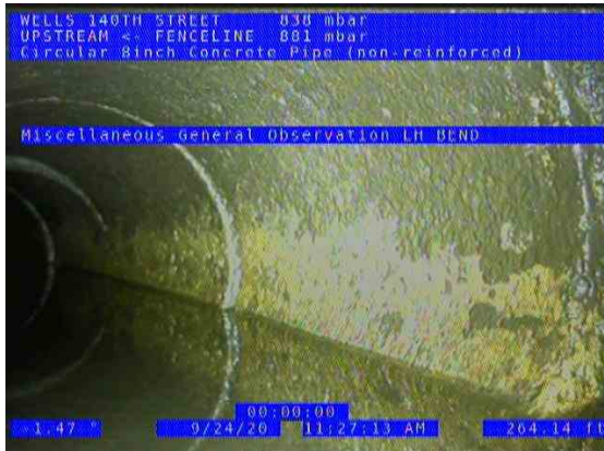
FENCELINE POINT (US) UPSTREAM_5cc3dc3c-849b-4201-92ed-bcc711c71ec7_2020 0924_114933_185.jpg, 00:07:15, 264.14ft Miscellaneous General Observation / LH BEND DEPTH 7' 5"
