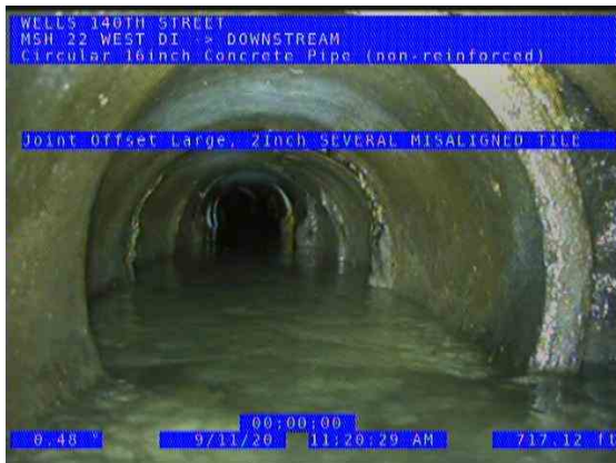
MSH 22 WEST DI (DS) DOWNSTREAM_1b0de49a-3c50-43ad-860d-2fce74c2a0fd_2 0200911_114056_027.jpg, 00:24:58, 717.12ft Joint Offset Large, 2Inch / SEVERAL MISALIGNED TILE
