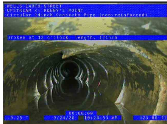
RONNY'S POINT (US) UPSTREAM_e629e8a9-806d-4c8b-93fc-dec3dc06f704_20200 924_105111_457.jpg, 00:17:52, 423.80ft Broken at 12 o'clock, length: 12inch
