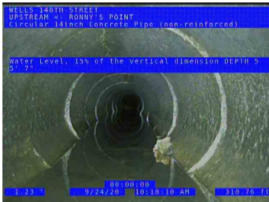
RONNY'S POINT (US) UPSTREAM_5205a8e1-407b-4426-a342-61df361cbd41_2020 0924_104028_489.jpg, 00:11:08, 310.76ft Water Level, 15% of the vertical dimension / DEPTH 5' 5" 7"
