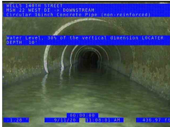
MSH 22 WEST DI (DS) DOWNSTREAM_ac0e8f26-a22d-484e-9e22-8cabbf0ae780_2 0200911_112829_153.jpg, 00:16:57, 436.97ft Water Level, 30% of the vertical dimension / LOCATER DEPTH 10'
