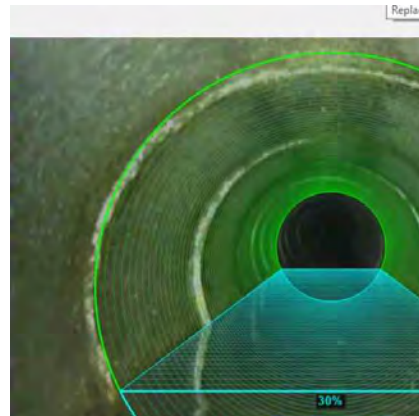
MSH 22 WEST (US) UPSTREAM_8bad4184-4052-46a6-bcb6-a0d48d365e20_202 00911_123038_955.jpg, 00:29:57, 597.75ft Water Level, 30% of the vertical dimension / LOCATER DEPTH
