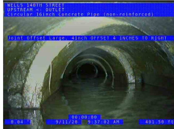
HUEPER BRANCH OUTLET (US) UPSTREAM_2a984b08-27c4-480c-8a30-1bf05978b7ae_20200911_095729_160.jpg, 00:14:18, 401.50ft Joint Offset Large, 4Inch / OFFSET 4 INCHES TO RIGHT
