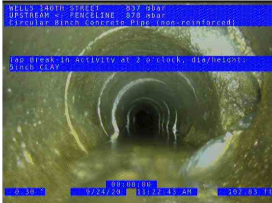
FENCELINE POINT (US) UPSTREAM_bd06800b-a3b2-49c1-b621-314e4227e21f_2020 0924_114502_201.jpg, 00:03:47, 102.83ft Tap Break-in Activity at 2 o'clock, dia/height: 5inch / CEMENT
