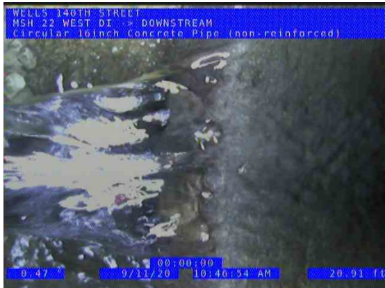
MSH 22 WEST DI (DS) DOWNSTREAM_33176324-8f5f-4e53-b5d2-2210f55fa073_20200911_110721_184.jpg, 00:02:11, 20.91ft Line Left Up, change to: 70% / CONCRETE
