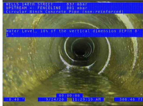
FENCELINE POINT (US) UPSTREAM_caf3f41d-e45d-4b4b-8a15-2331daf04ce6_2020 924_115139_245.jpg, 00:08:47, 306.46ft Water Level, 10% of the vertical dimension / DEPTH 8' 3 "
