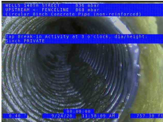
FENCELINE POINT (US) UPSTREAM_0d8b17d8-129b-4b6f-a301-59098cd11c0c_2020 0924_122028_542.jpg, 00:26:06, 757.30ft Tap Break-in Activity at 3 o'clock, dia/height: 5inch / PRIVATE
