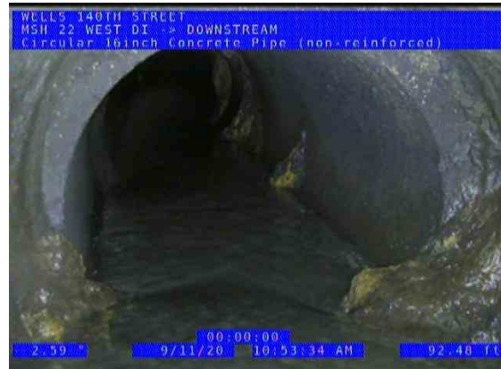
MSH 22 WEST DI (DS) DOWNSTREAM_4c92aa14-10ef-4d35-b7b0-b0a79ce63b28_2 0200911_111400_919.jpg, 00:07:45, 92.48ft Miscellaneous Material Change / END OF CMP UNDER MSH 22
