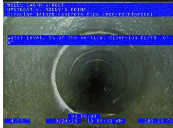
RONNY'S POINT (US) UPSTREAM_9bcee977-fada-4dd3-94db-8d8cf2e44f8f_2020 924_103214_010.jpg, 00:06:20, 165.25ft Water Level, 5% of the vertical dimension / DEPTH 6' 6"
