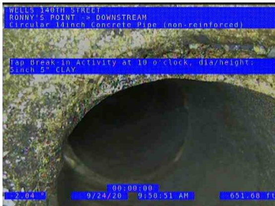
RONNY'S POINT (DS) DOWNSTREAM_17c21c9d-e368-4a52-931d-e44d33640a13_ 20200924_101309_203.jpg, 00:15:30, 651.68ft Tap Break-in Activity at 10 o'clock, dia/height: 5inch / 5" CLAY
