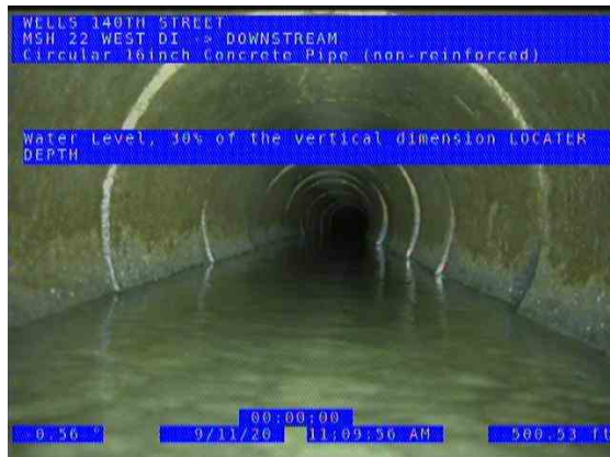
MSH 22 WEST DI (DS) DOWNSTREAM_808e009f-0061-494d-9953-a43c3b84d83a_2 0200911_113022_945.jpg, 00:18:12, 500.53ft Water Level, 30% of the vertical dimension / LOCATER DEPTH
