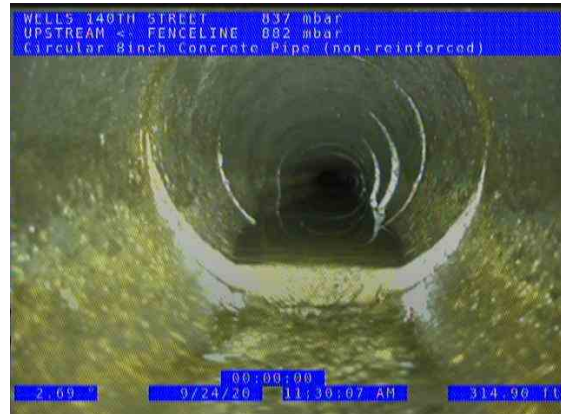
FENCELINE POINT (US) UPSTREAM_d19612e0-6dd7-4217-826c-3bd70d86f5e1_2020 0924_115226_949.jpg, 00:09:00, 311.79ft Water Level, 5% of the vertical dimension / HUMP IN PIPE
