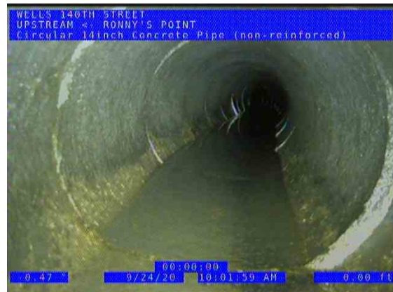
RONNY'S POINT (US) UPSTREAM_fcb3e791-adb1-481f-b8da-6ae5d68040c6_2020 0924_102417_239.jpg, 00:00:07, 0.00ft Water Level, 5% of the vertical dimension
