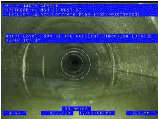
MSH 22 WEST (US) UPSTREAM_7694e5a2-c69b-4aec-bdc1-2e674d9b5b1f_2020 0911_122832_374.jpg, 00:29:57, 498.96ft Water Level, 50% of the vertical dimension / LOCATER DEPTH 10' 1"
