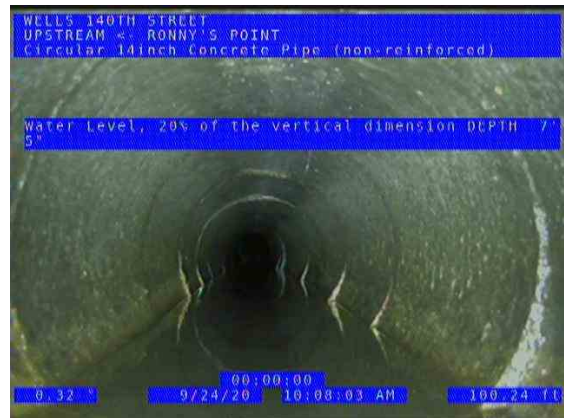
RONNY'S POINT (US) UPSTREAM_9425705f-d2ae-4d64-bcb2-1022bf8bfe16_20200 924_103021_693.jpg, 00:05:09, 100.24ft Water Level, 20% of the vertical dimension / DEPTH 7' 5"
