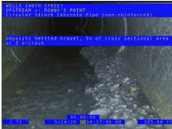
RONNY'S POINT (US) UPSTREAM_1df92873-2d35-4379-af25-858b25836c2d_2020 0924_103923_835.jpg, 00:10:45, 305.00ft Deposits Settled Gravel, 5% of cross sectional area at 5 o'clock
