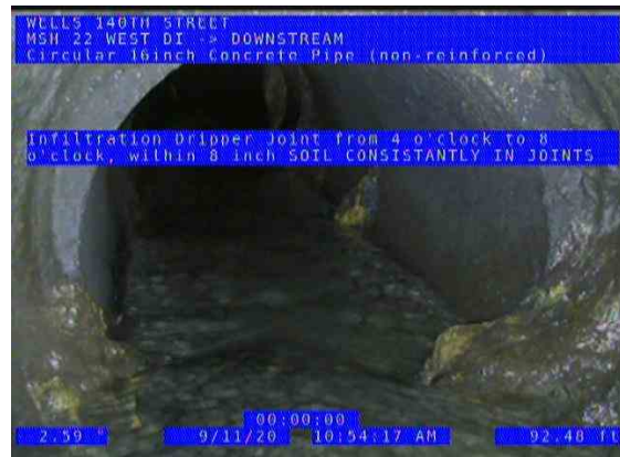
MSH 22 WEST DI (DS) DOWNSTREAM_8b752099-743d-4bde-b97f-68672c156f28_2 0200911_111444_739.jpg, 00:07:57, 92.48ft Infiltration Dripper Joint from 4 o'clock to 8 o'clock, within 8 inch / SOIL CONSISTANTLY IN JOINTS
