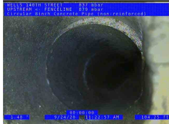
FENCELINE POINT (US) UPSTREAM_cd41253a-83c5-4676-bb6e-82c7940ec7f4_2020 0924_114516_747.jpg, 00:03:47, 102.83ft Tap Break-in Activity at 2 o'clock, dia/height: 5inch / CEMENT
