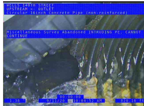
HUEPER BRANCH OUTLET (US) UPSTREAM_3efdb1d3-9e10-4ad2-b597-5755230bc17f_2020 0911_102519_138.jpg, 00:30:55, 820.16ft Miscellaneous Survey Abandoned / INTRUDING PE, CANNOT CONTINUE
