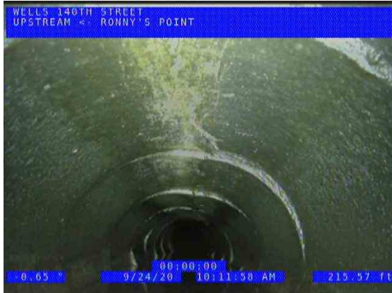
RONNY'S POINT (US) UPSTREAM_ed7e8834-2e4d-4ab5-af6f-208567e58228_2020 0924_103416_527.jpg, 00:07:24, 215.57ft Crack Longitudinal at 12 o'clock / STARTS
