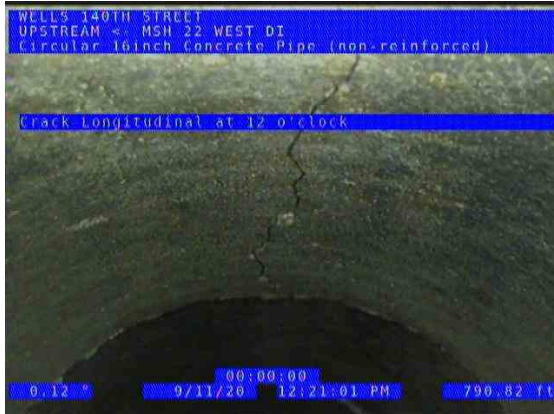
MSH 22 WEST (US) UPSTREAM_b4fc8e30-b879-4f3c-8cbe-e9c28bfa50c6_20200911_124128_599.jpg, 00:29:57, 790.82ft Crack Longitudinal at 12 o'clock
