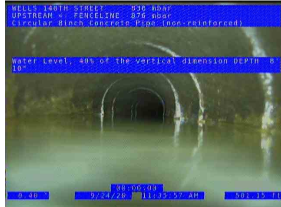
FENCELINE POINT (US) UPSTREAM_6821c268-038e-417e-9a25-d38b031e7b0e_202 00924_115816_223.jpg, 00:13:01, 501.15ft Water Level, 40% of the vertical dimension / DEPTH 8' 10"
