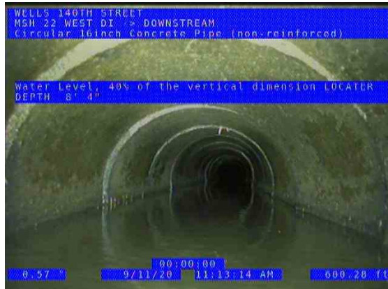
MSH 22 WEST DI (DS) DOWNSTREAM_c106f42c-75e0-4119-9c7e-4848ae146b94_2 0200911_113342_367.jpg, 00:20:21, 600.28ft Water Level, 40% of the vertical dimension / LOCATER DEPTH 8' 4"
