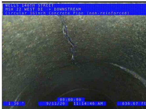
MSH 22 WEST DI (DS) DOWNSTREAM_a5d005bb-fe03-467a-9310-f0a8782cfb82_2 0200911_113514_004.jpg, 00:21:20, 632.72ft Broken at 12 o'clock, length: 1inch / 2 BROKEN TILE LOCATER DEPTH 8' 2"
