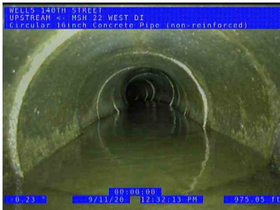
MSH 22 WEST (US) UPSTREAM_961ca001-1351-45cf-98e5-e8cb173609e4_2020 0911_125239_766.jpg, 00:29:57, 975.04ft Water Level, 35% of the vertical dimension / LOCATER DEPTH 9' 7"
