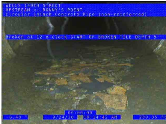
RONNY'S POINT (US) UPSTREAM_39a809de-0ae9-4101-a0b9-3fa7217bcde0_2020 0924_103700_818.jpg, 00:09:24, 289.35ft Broken at 12 o'clock / START OF BROKEN TILE DEPTH 5' 9"
