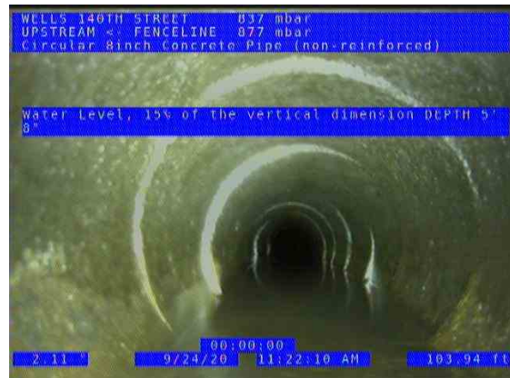
FENCELINE POINT (US) UPSTREAM_750ce619-4ff4-47f7-b6a3-eabacdbfeec3_20200 924_114429_321.jpg, 00:03:36, 103.94ft Water Level, 15% of the vertical dimension / DEPTH 5' 8"
