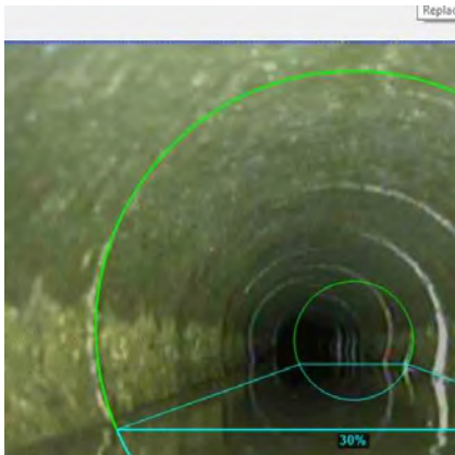
FENCELINE POINT (US) UPSTREAM_6b851c5d-c45c-4851-a6b1-b379e17d4a5c_2020 0924_120415_265.jpg, 00:17:52, 701.16ft Water Level, 30% of the vertical dimension / DEPTH 6' 8"
