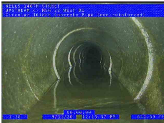
MSH 22 WEST (US) UPSTREAM_7cc917a1-7919-4a3e-9972-5ae500c03969_20200911_123403_798.jpg, 00:29:57, 638.61ft Joint Offset Large, 2Inch / 9.7% OBSTRUCTED
