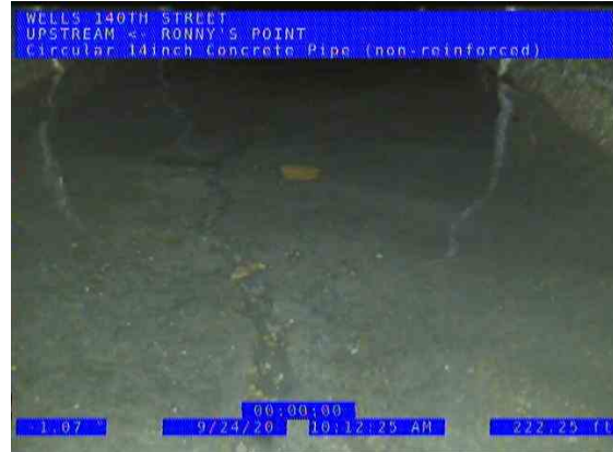
RONNY'S POINT (US) UPSTREAM_a178090c-a63a-4ab7-af60-a3e73fa6efc3_2020 0924_103443_442.jpg, 00:07:24, 215.57ft Crack Longitudinal at 12 o'clock / STARTS
