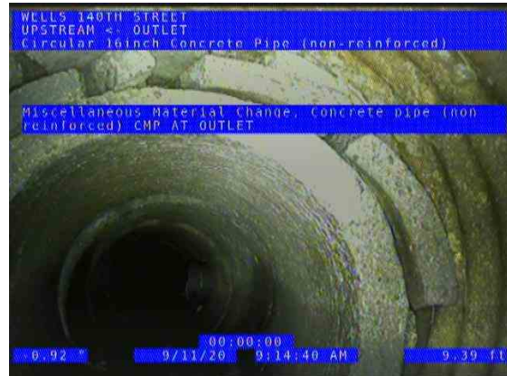
HUEPER BRANCH OUTLET (US) UPSTREAM_a0409254-b129-4b20-bdd1-06134a1efa4b_2020 0911_093508_397.jpg, 00:00:51, 9.39ft Miscellaneous Material Change, Concrete pipe (non reinforced) / CMP AT OUTLET
