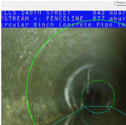
FENCELINE POINT (US) UPSTREAM_14bafc3d-84ef-46d8-98e7-6c73e8b4929c_2020 0924_121357_384.jpg, 00:25:39, 970.39ft Water Level, 20% of the vertical dimension / DEPTH 4" 3"
