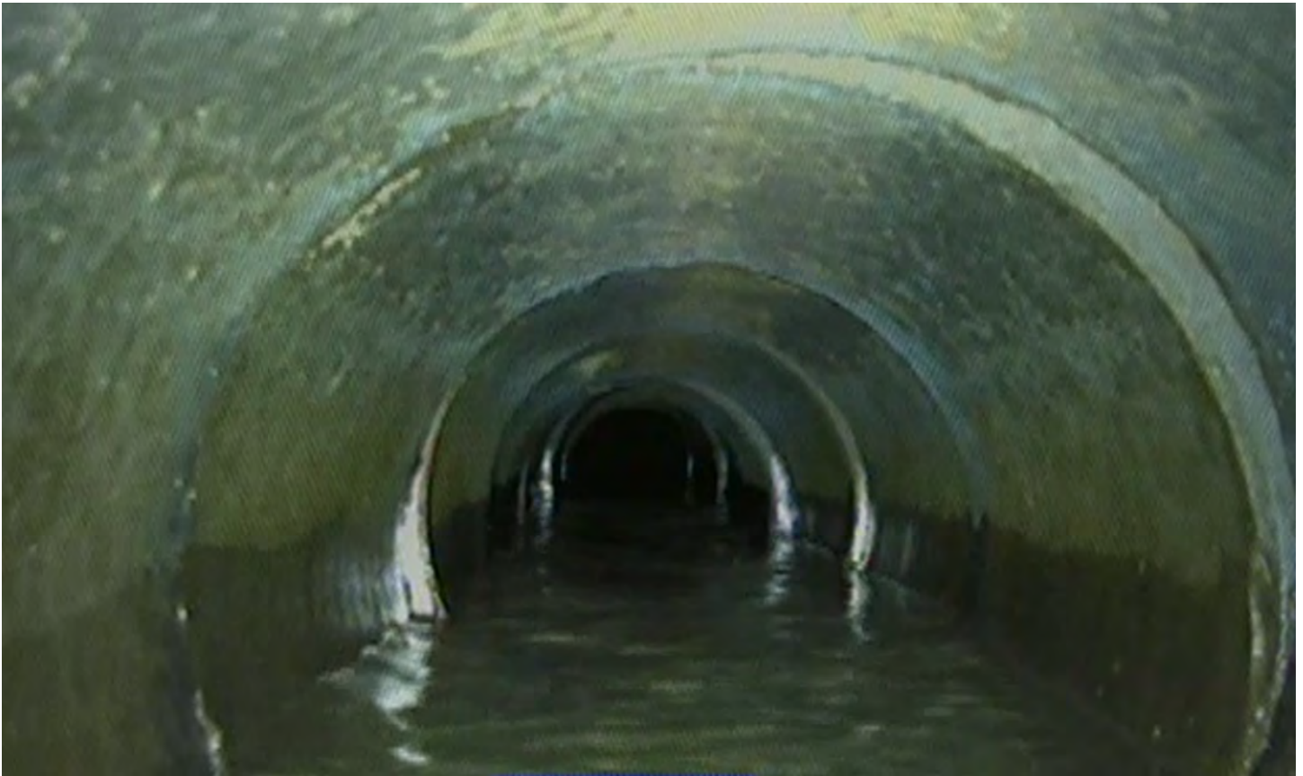
Figure 16: Televising at the Tile Outlet into Open Ditch
