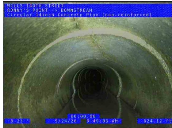
RONNY'S POINT (DS) DOWNSTREAM_ee76ac7b-b14f-43b8-98d4-fd27049e56e5_2 0200924_101124_515.jpg, 00:14:31, 624.12ft Crack Longitudinal at 1 o'clock
