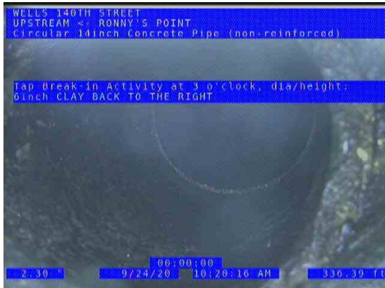
RONNY'S POINT (US) UPSTREAM_25a97eac-e7c5-498a-b782-ec34f1a1fbfa_20200924_104234_763.jpg, 00:12:16, 336.39ft Tap Break-in Activity at 3 o'clock, dia/height: 6inch / CLAY BACK TO THE RIGHT
