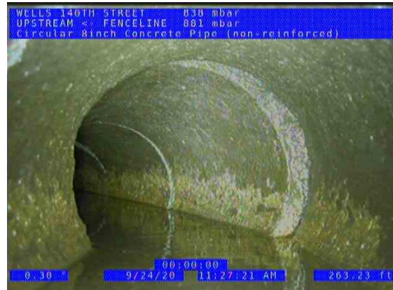
FENCELINE POINT (US) UPSTREAM_c6b030dd-a1bf-4760-a5f3-7ef85b69e781_2020 924_114941_752.jpg, 00:07:15, 264.14ft Miscellaneous General Observation / LH BEND DEPTH 7' 5"
