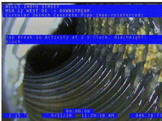
MSH 22 WEST DI (DS) DOWNSTREAM_3228d2a5-0b44-48cc-b0c3-b5825887554a_20200911_114836_497.jpg, 00:29:12, 846.78ft Tap Break-in Activity at 2 o'clock, dia/height: 6inch
