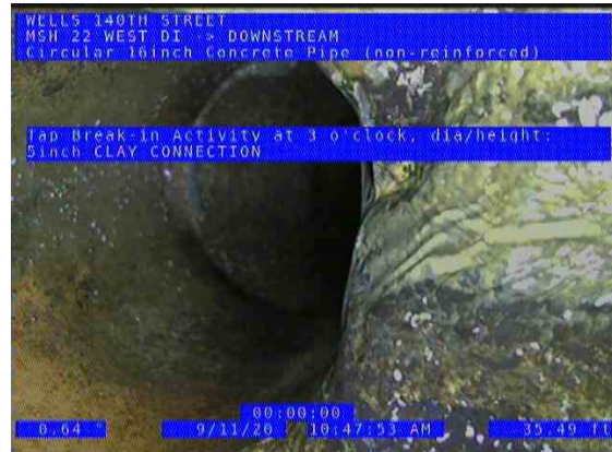
MSH 22 WEST DI (DS) DOWNSTREAM_db00fba8-2ea8-44e9-8324-38796641c0a0_20200911_110819_870.jpg, 00:03:09, 35.49ft Tap Break-in Activity at 3 o'clock, dia/height: 5inch / CLAY CONNECTION
