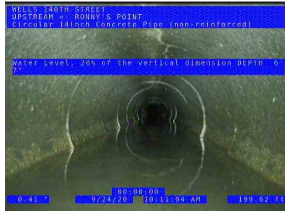
RONNY'S POINT (US) UPSTREAM_21c49a0a-b7d8-4f46-8a9f-84ab6851bb36_202 0924_103322_949.jpg, 00:06:54, 199.62ft Water Level, 20% of the vertical dimension / DEPTH 6' 7"
