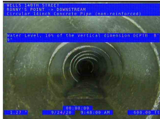
RONNY'S POINT (DS) DOWNSTREAM_76e63014-4edf-4001-b94f-69e66203887c_2 0200924_101019_145.jpg, 00:13:39, 600.00ft Water Level, 10% of the vertical dimension / DEPTH 8' 9"
