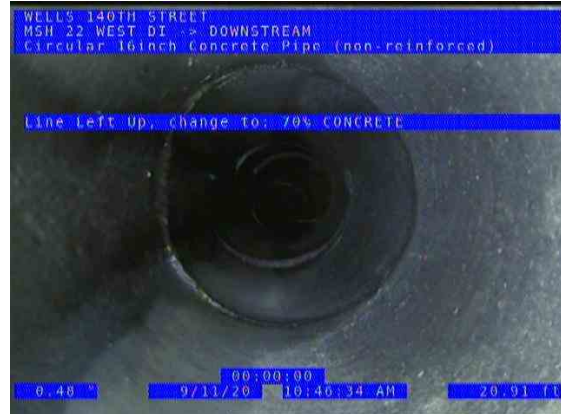
MSH 22 WEST DI (DS) DOWNSTREAM_2db46f63-ece5-451b-8f3c-84c46c1d92f8_20200911_110702_056.jpg, 00:02:11, 20.91ft Line Left Up, change to: 70% / CONCRETE
