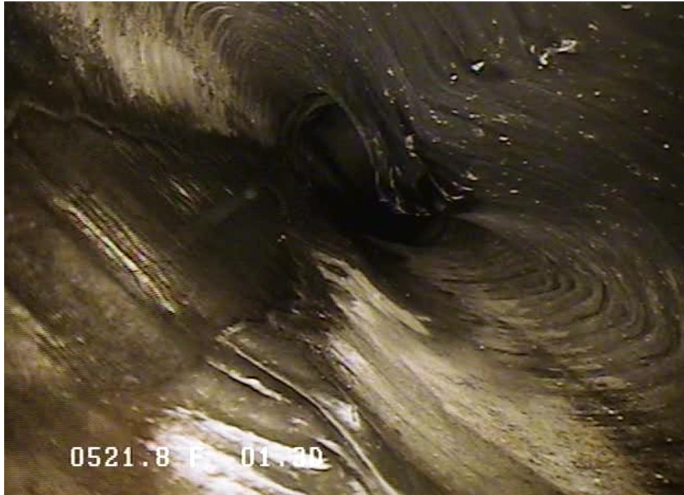
Figure 7. Completely Collapsed Tile. (Just South of Impulse Road)
