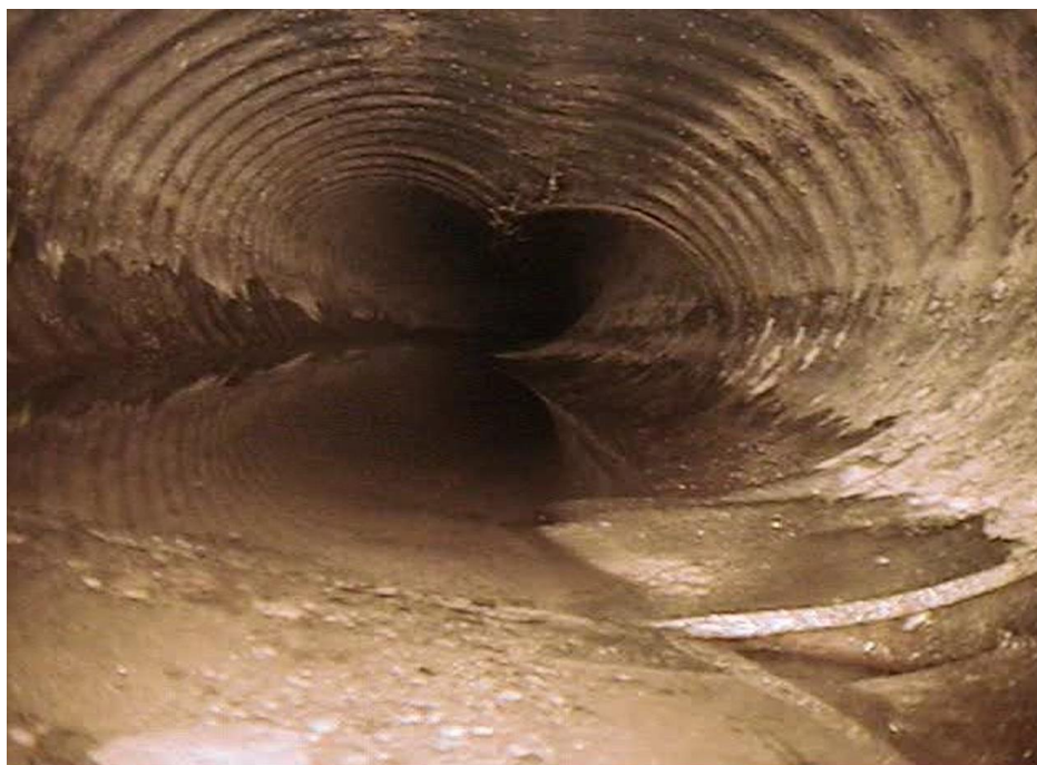
Figure 3. Oval Shape, Cracks on Top
