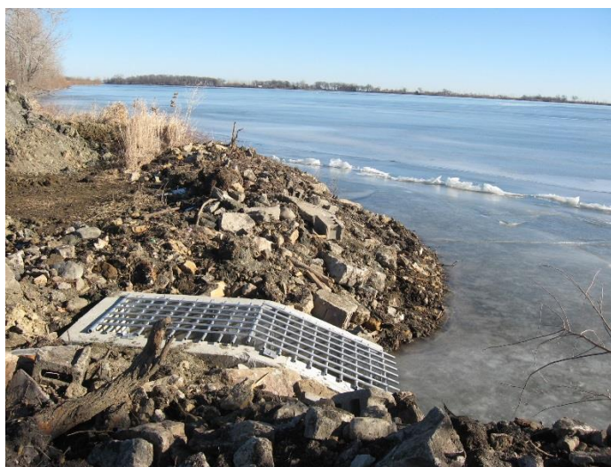
Figure 1. Installed New Outlet Structure
