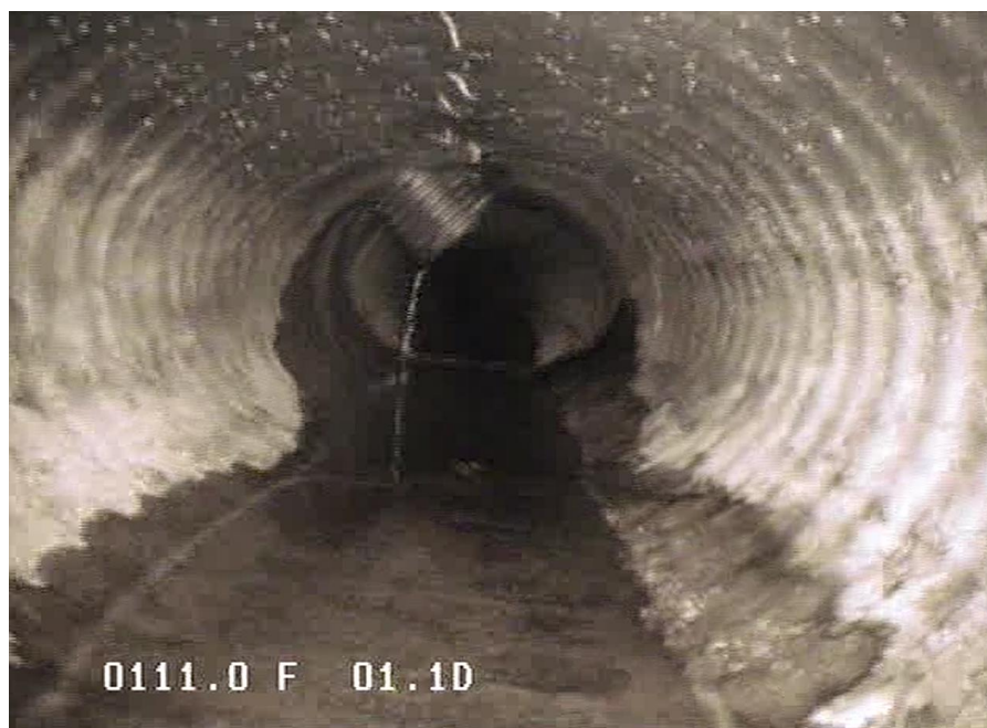
Figure 4. Intruding Tile Restricting Flow
