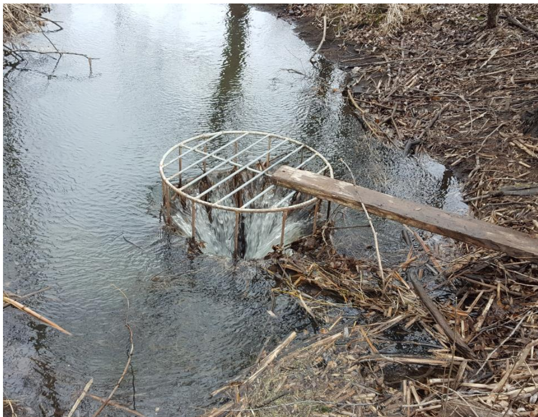
Figure 8. 30-Inch DNR Drop Intake Structure
