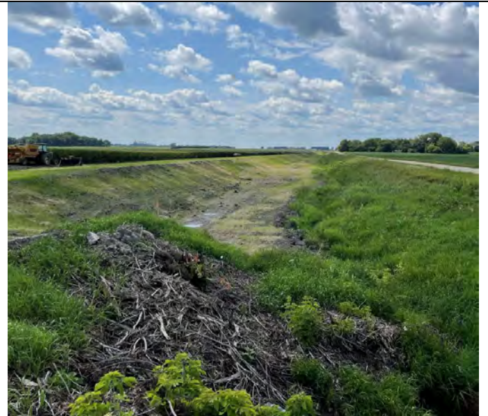
Constructed Two-Stage Ditch
