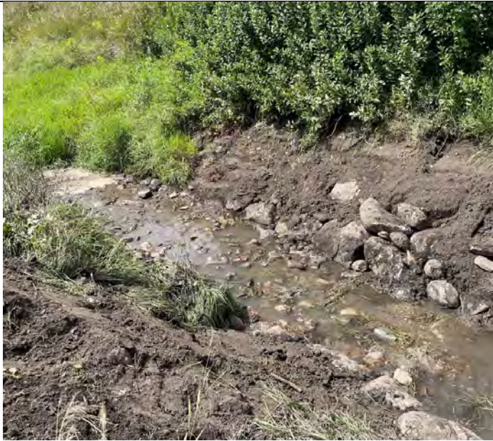
Installed Rock Riffle Structure
