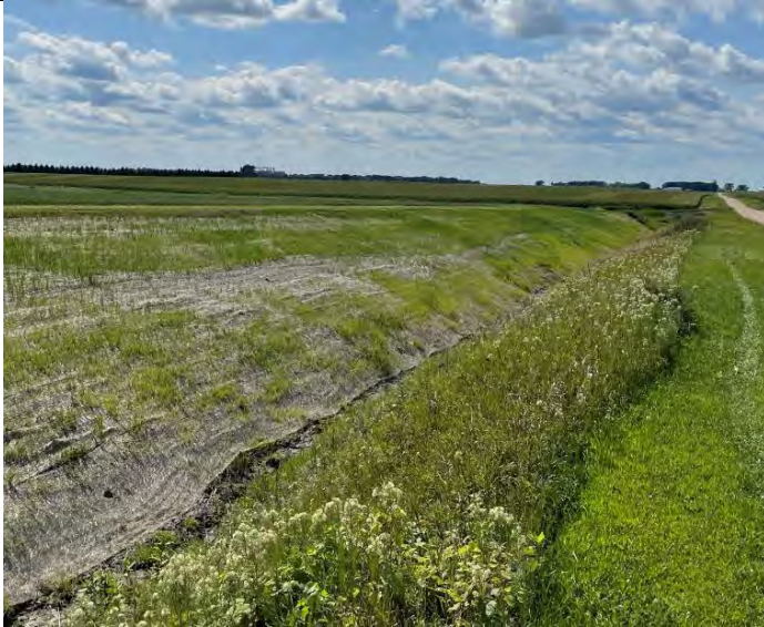
Outlet Sideslope flattening
