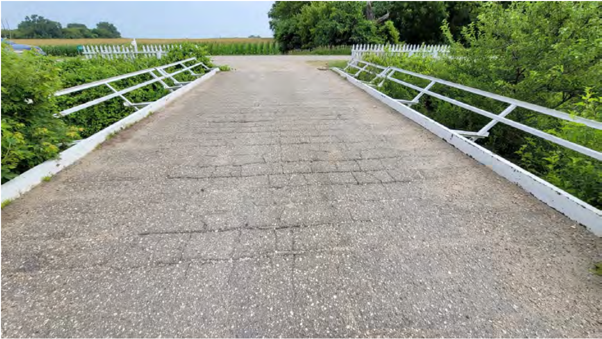
Figure 7. Paved Decking Beginning to Crack and Separate
