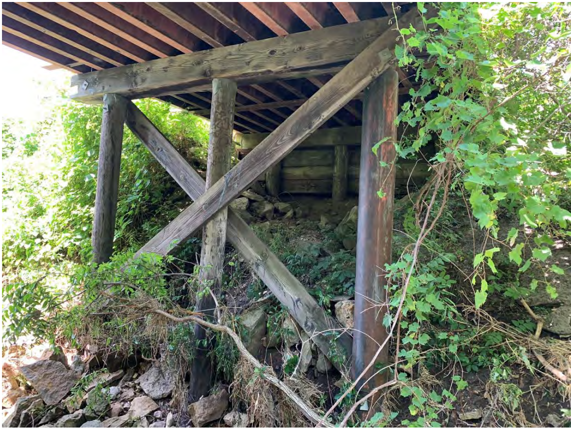
Figure 4. Timber Bridge Supports and Cross Members
