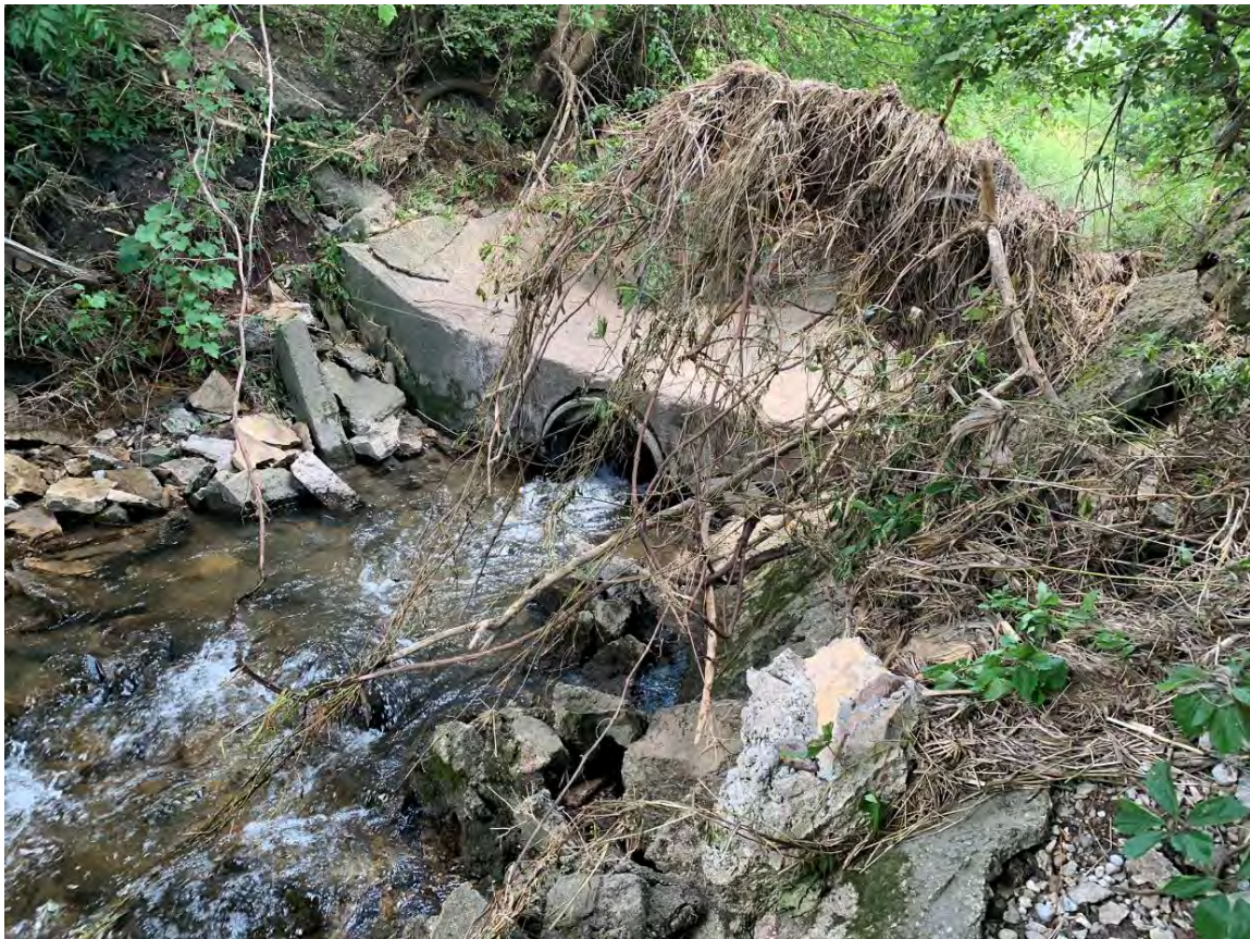
Figure 5. Concrete Base-Flow Grade Control Structure
