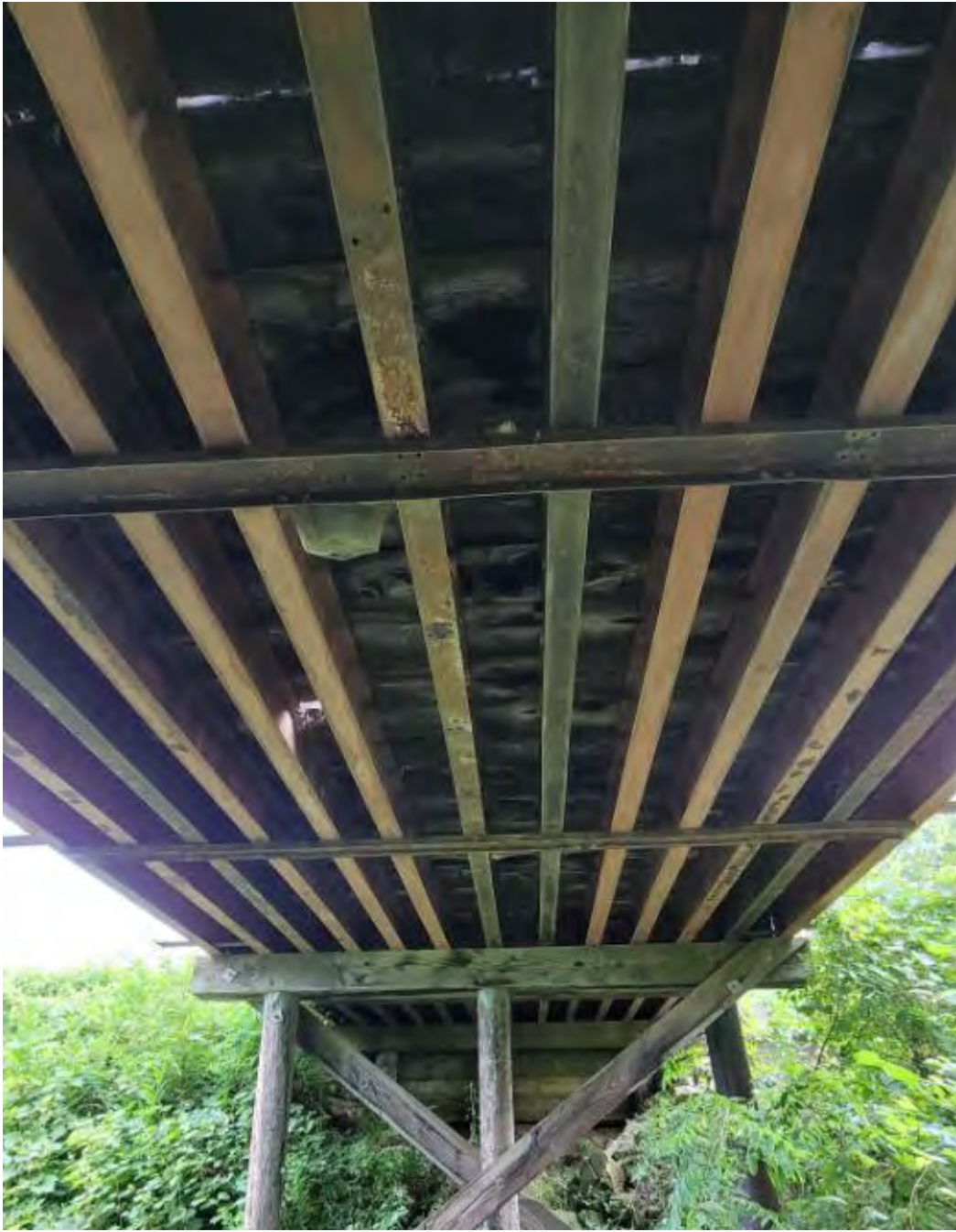
Figure 6. Steel Span Beams and Timber Decking, Gaps and Voids in Decking
