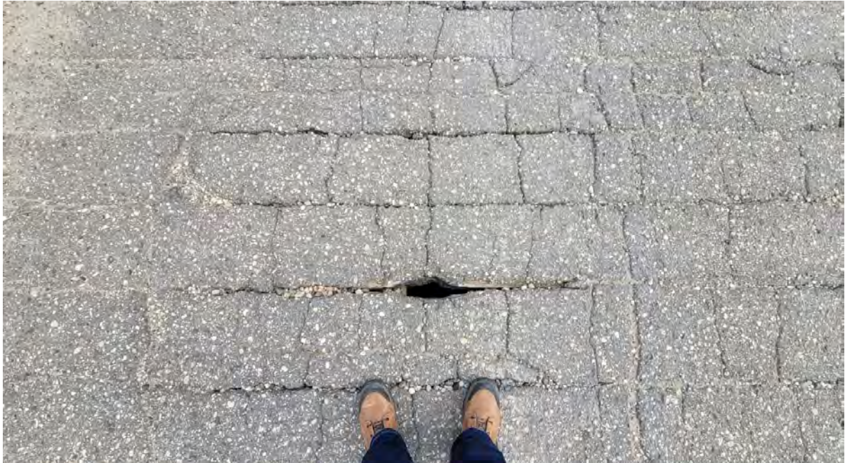
Figure 8. Gaps and Voids Arising on Driving Surface
