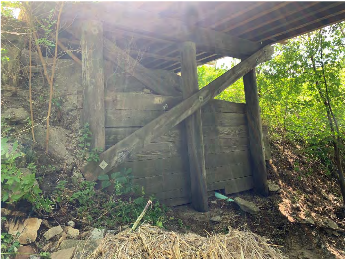
Figure 3. Bridge Supports and Timber Wing/Retaining Wall
