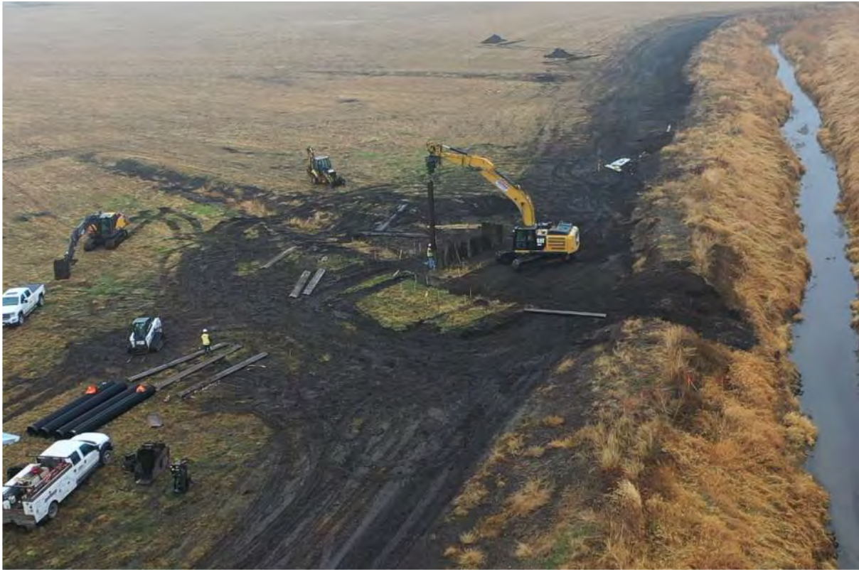
Wetland outlet sheet pile installation
