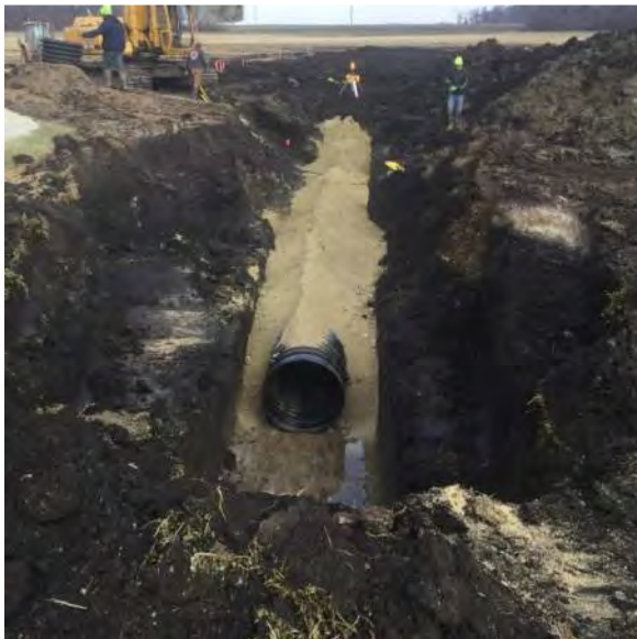
Typical Leland Ag Tile Installation
