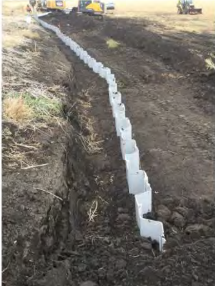
Typical vinyl sheet pile installation
