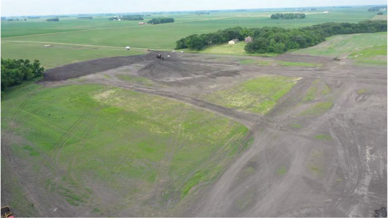
Wetland Excavation at Branch S Tile outlet
