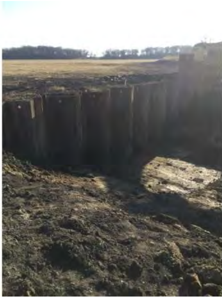
Weir installation prior to rip rap
