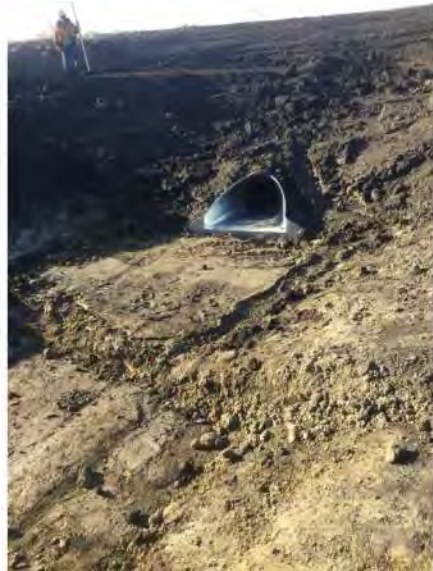
Inlet downstream of weir
