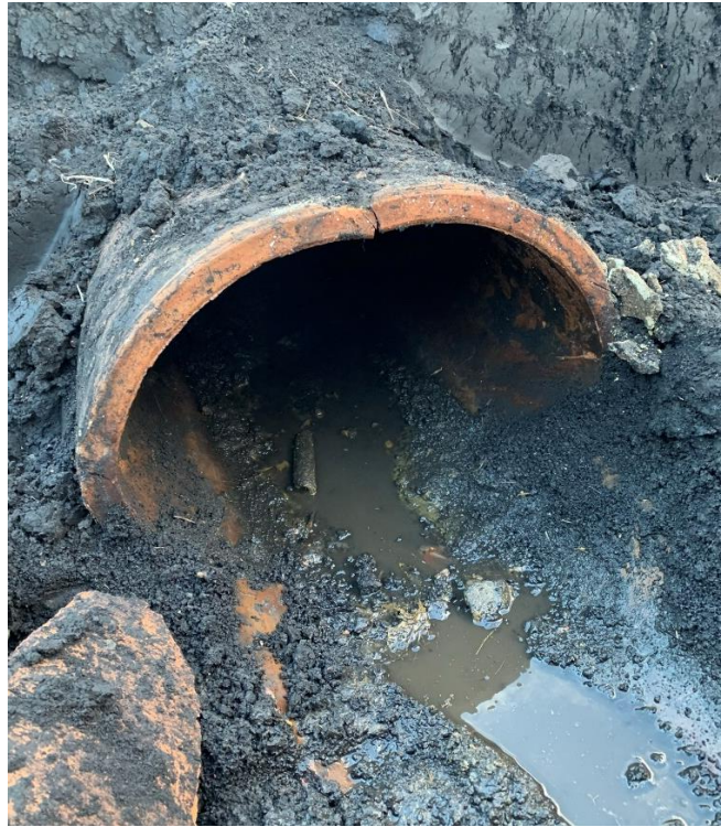
Figure 1. Excavation of the East Main and televising showed that the tile is out of repair. Cracked tile and sediment accumulation prevented a full investigation of the tile.
