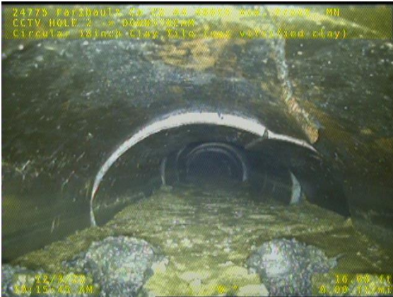
Figure 1. Excavation of the East Main and televising showed that the tile is out of repair. Cracked tile and sediment accumulation prevented a full investigation of the tile.
