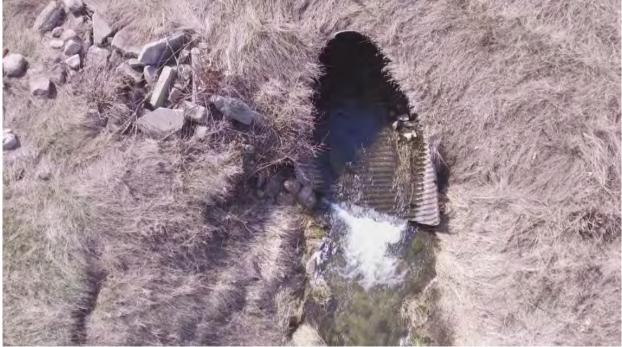
Figure 19: Culvert set above ditch grade on CSAH 19
