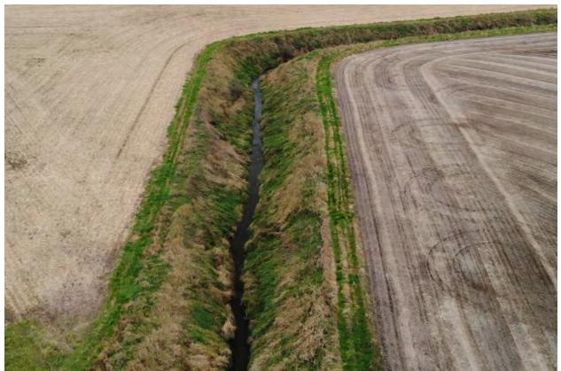
*Figure 29: Tall Banks and Deep Excavation Requiring Side Slope Flattening in Section 13 of Barber Township*
