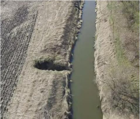
Figure 17: Washout in the NE ¼ of Section 16 Lura Township
