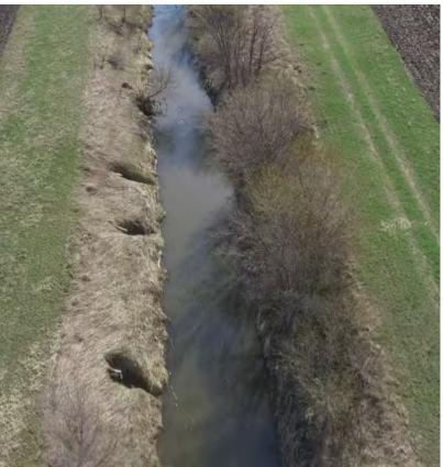
Figure 13. Unprotected Tile in the SW ¼ of Section 15 Lura Township
