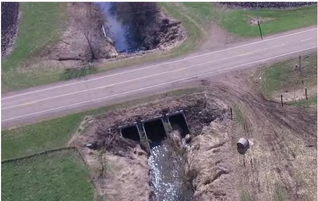
Figure 18: Box Culverts filled with sediment on CSAH 17
