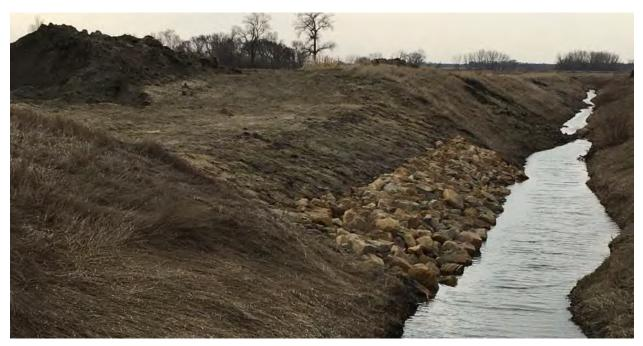
Figure 27: Repaired Slough with Bench Slope
