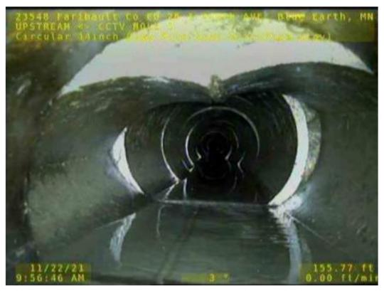
Figure 13. Collapsing Tile (Station 99+00)
