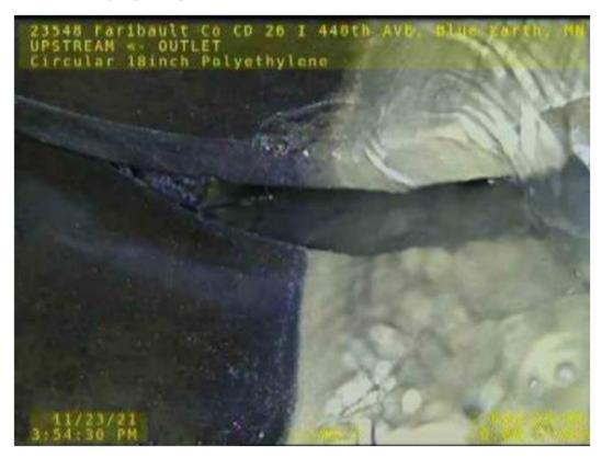
Figure 4. Misalignment in Tile Sections (Station 5+10)
