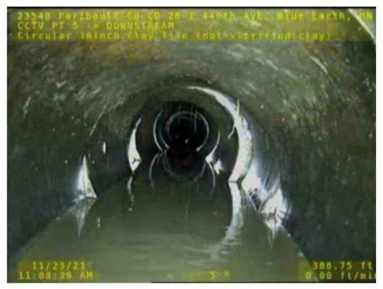
Figure 7. Misalignment in Tile Sections (Station 40+10)
