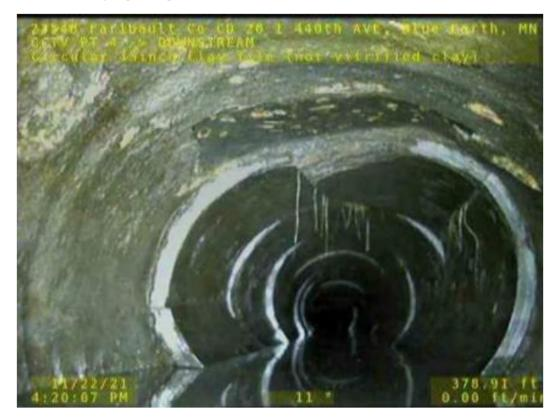
Figure 10. Collapsing Tile & Root Intrusion (Station 72+25)
