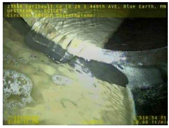
Figure 3. Misalignment in Tile Sections (Station 5+10)
