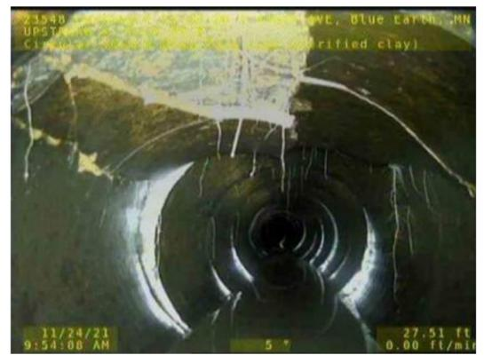
Figure 5. Collapsing Tile & Root Intrusion (Station 5+25)
