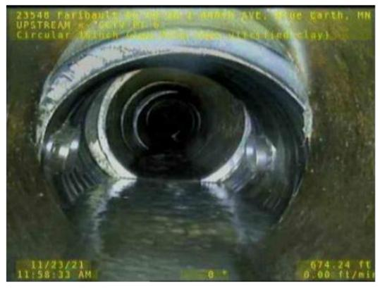
Figure 9. Deflection in Dual Wall Patch (Station 58+75)
