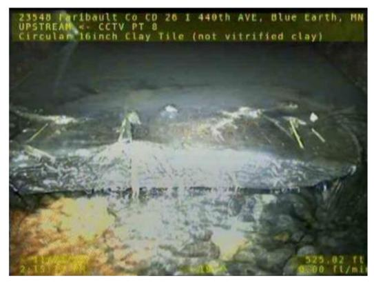
Figure 11. Tile Chunk Obstruction (Station 73+25)
