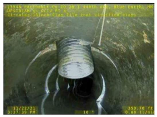
Figure 12. Connection Blocking Flow (Station 79+75)
