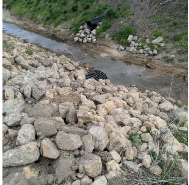
Branch 275 Outlet with Rip Rap overflow (near) and Typical tile outlet (across ditch)
