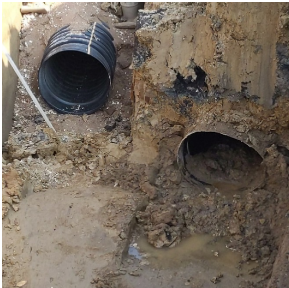
Connection point for re-route of tile. Crushing of original install is clear.
