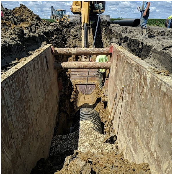
Trench box used for safe installation of tile re-route. Spooned bottom tile installation is being used.
