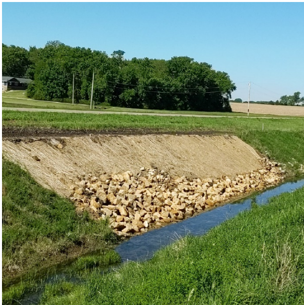
Typical slough repair with Rip Rap Toe stabilization and side slope seeding with MnDOT erosion control blanket.
