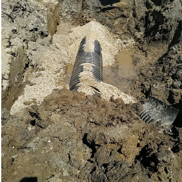
New tile spliced into existing line. Bedded and completely encased in rock.
