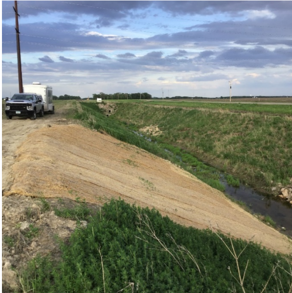
Typical slough repair with side slope seeding with MnDOT erosion control blanket.
