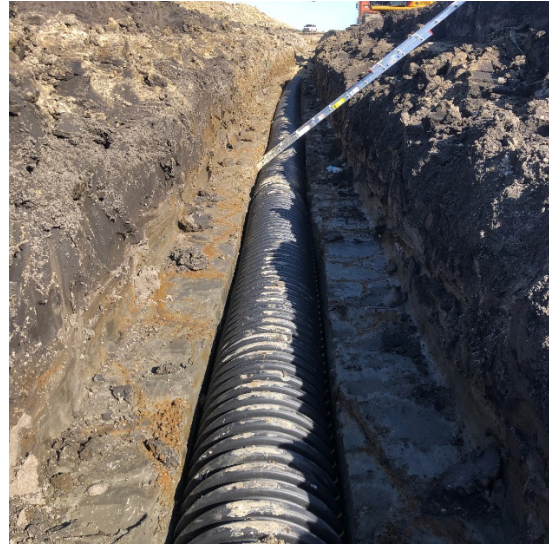
Typical tile installation with the spoon trench method.
