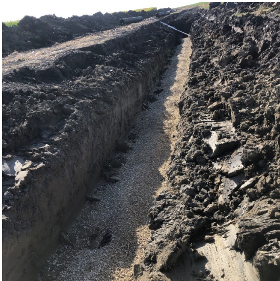
Installed tile was backfilled with rock granular material.
