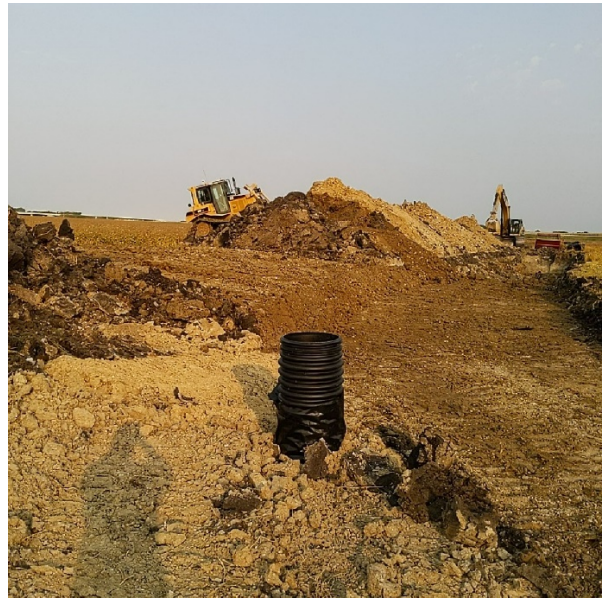
Drop intake was replaced, wrapped in fabric, and backfilled per specifications.
