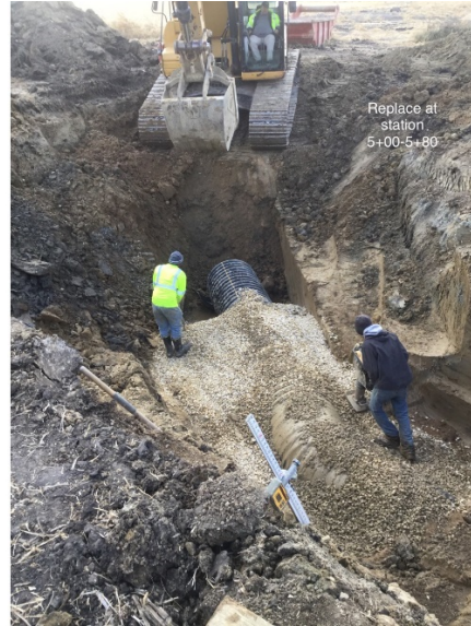
Typical tile installation with flat bottom trench and granular backfill. Rock used around all fittings.
