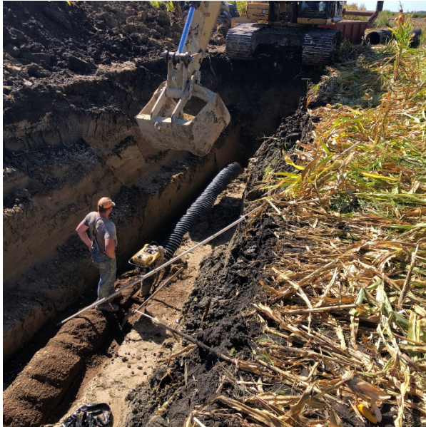
Typical tile installation with flat bottom trench and compacted granular backfill.
