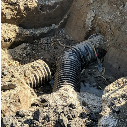
New tile was connected to existing HDPE tile for reroute repair.
