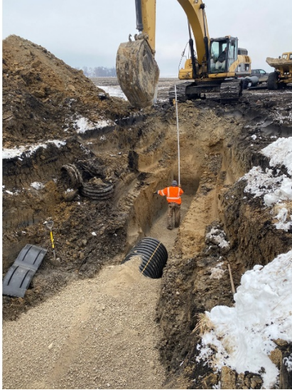
Typical tile installation with flat bottom trench and granular backfill.
