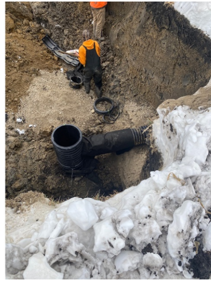
Installed drop intake and connected existing tile line into it.
