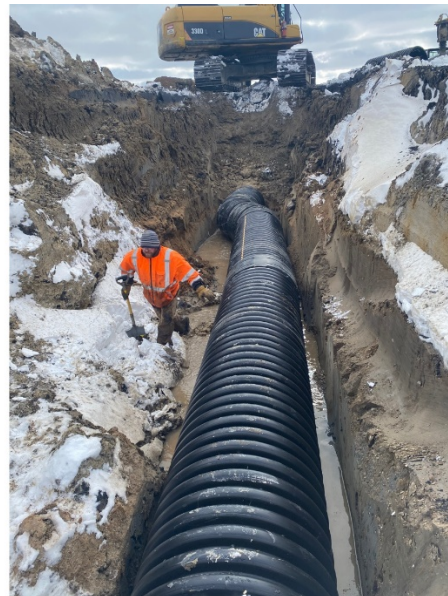
Connected to existing HDPE tile with multiple prefabricated bends.
