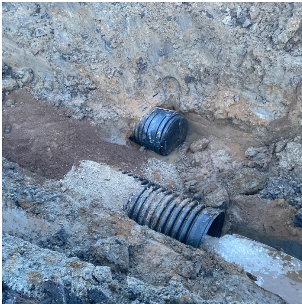
Existing HDPE tile line was capped and abandoned.
