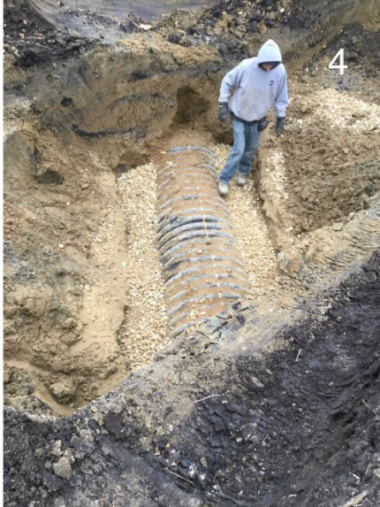
Deflections repaired by releasing pressure from tile and compacting rock along the sides to support pipe.
