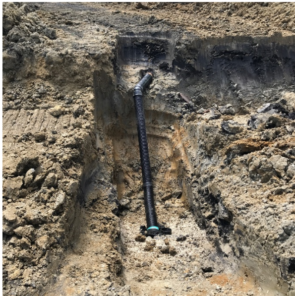
Private tile connection made with dual wall, HDPE pipe.
