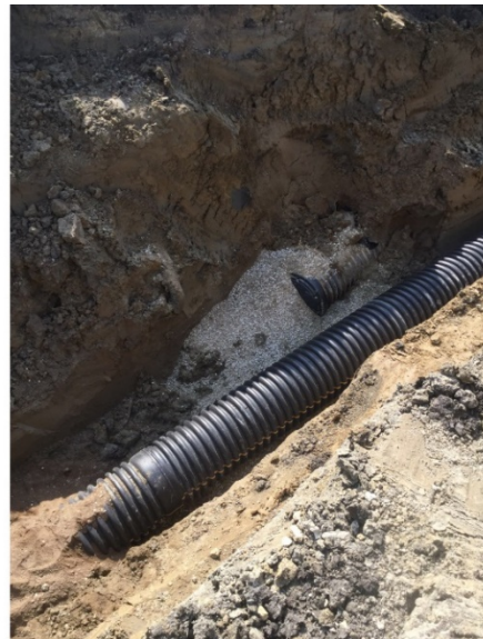
New installation of Branch 275. Existing HDPE line was capped and encased in rock.
