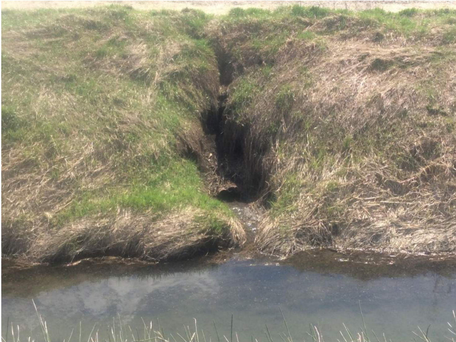
Field Survey Photograph 5: Erosion and Side Inlet at Station 45+50
