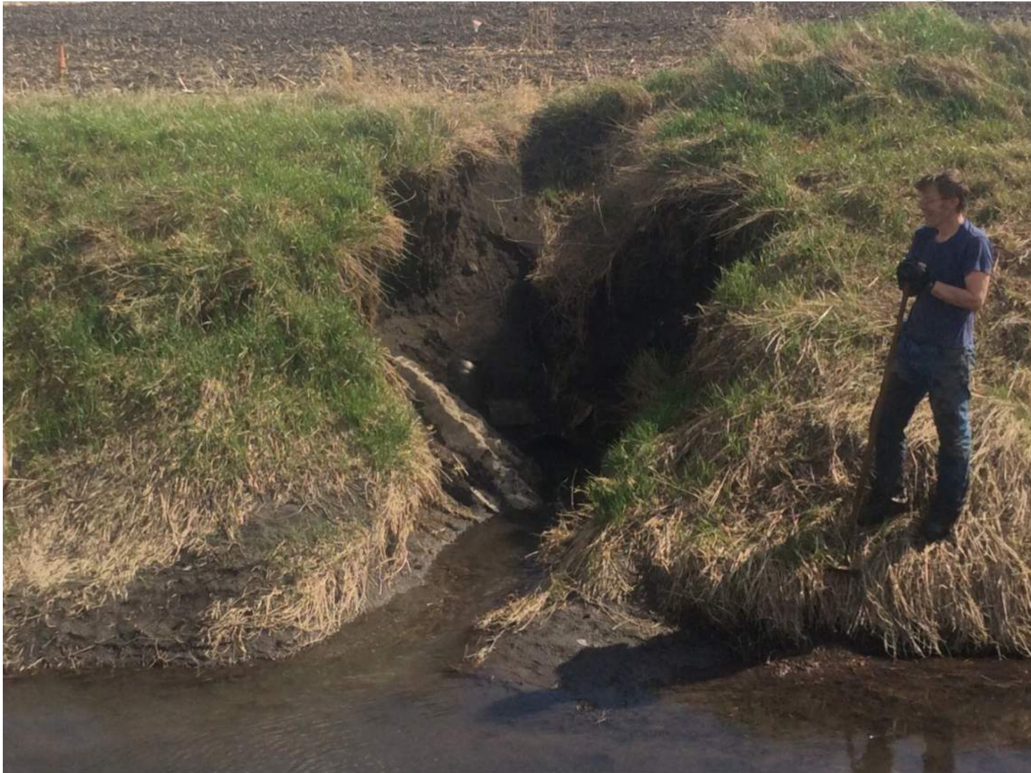
Field Survey Photograph 7: 12" RCP Drain tile Outlet and Eroded Bank at Station 100+00
