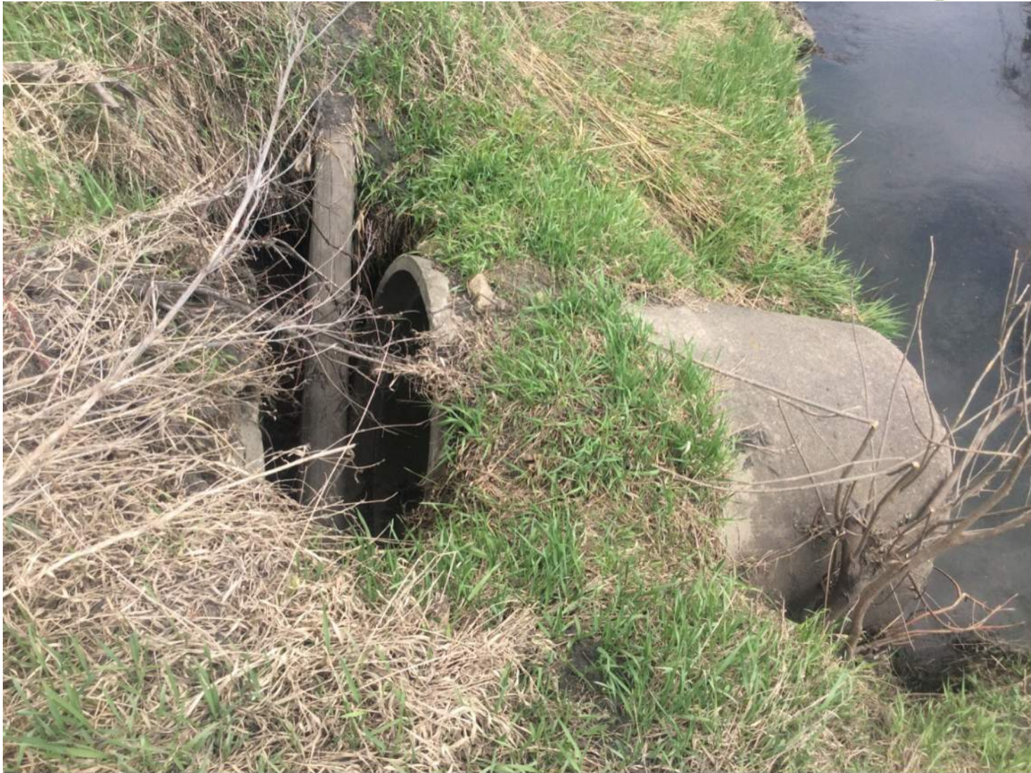
Field Survey Photograph 6: Broken 42" RCP at Station 69+00
