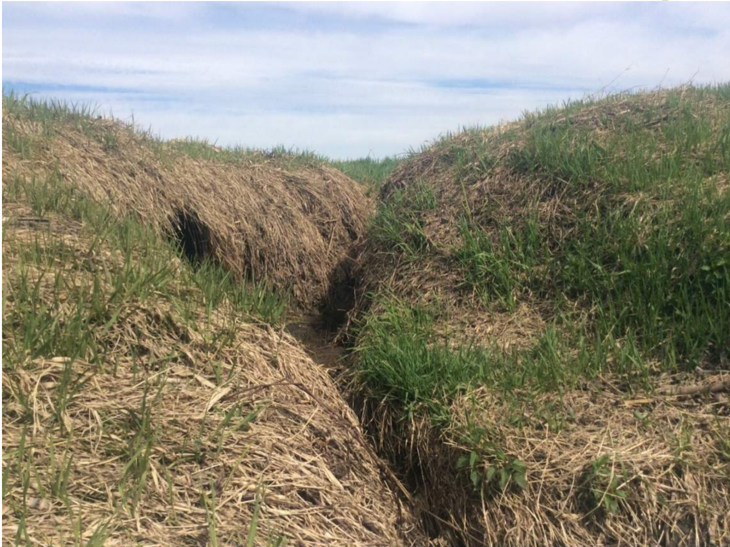
Field Survey Photograph 4: Eroded Bank at Station 30+00
