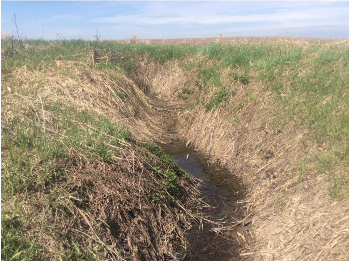
Field Survey Photograph 1: Eroded Bank at Station 6+00
