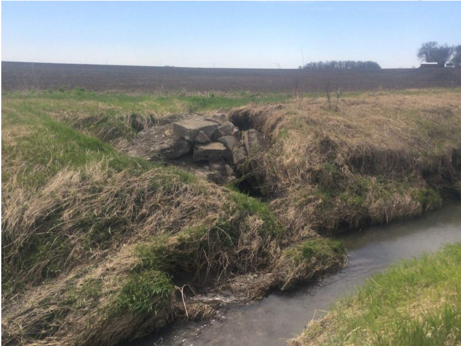
Field Survey Photograph 2: Eroded Bank and Fill at Station 10+50
